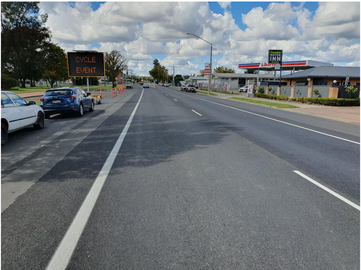
Finished surface Glen Innes Road
