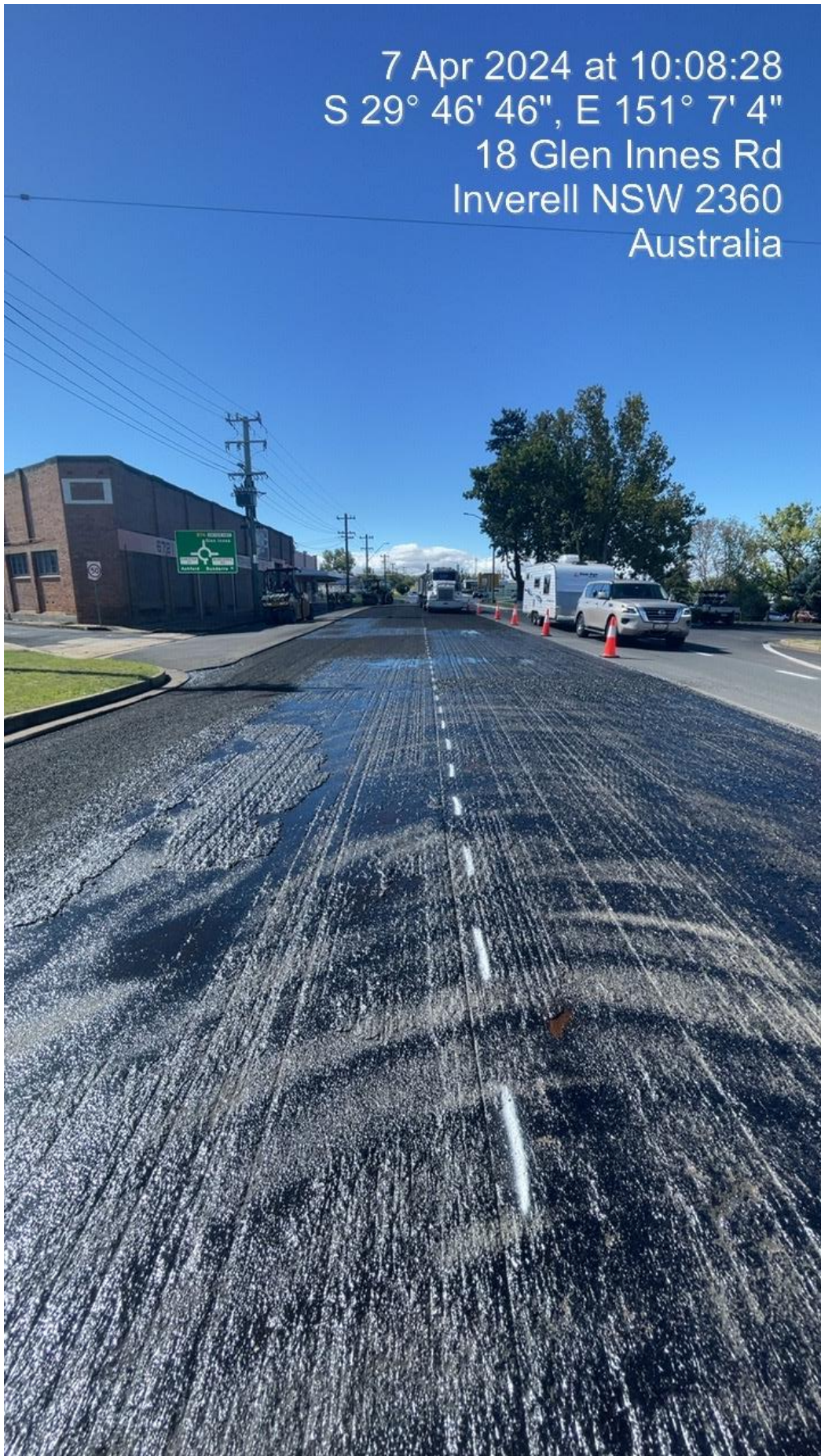
Asphalt Preparation Works
