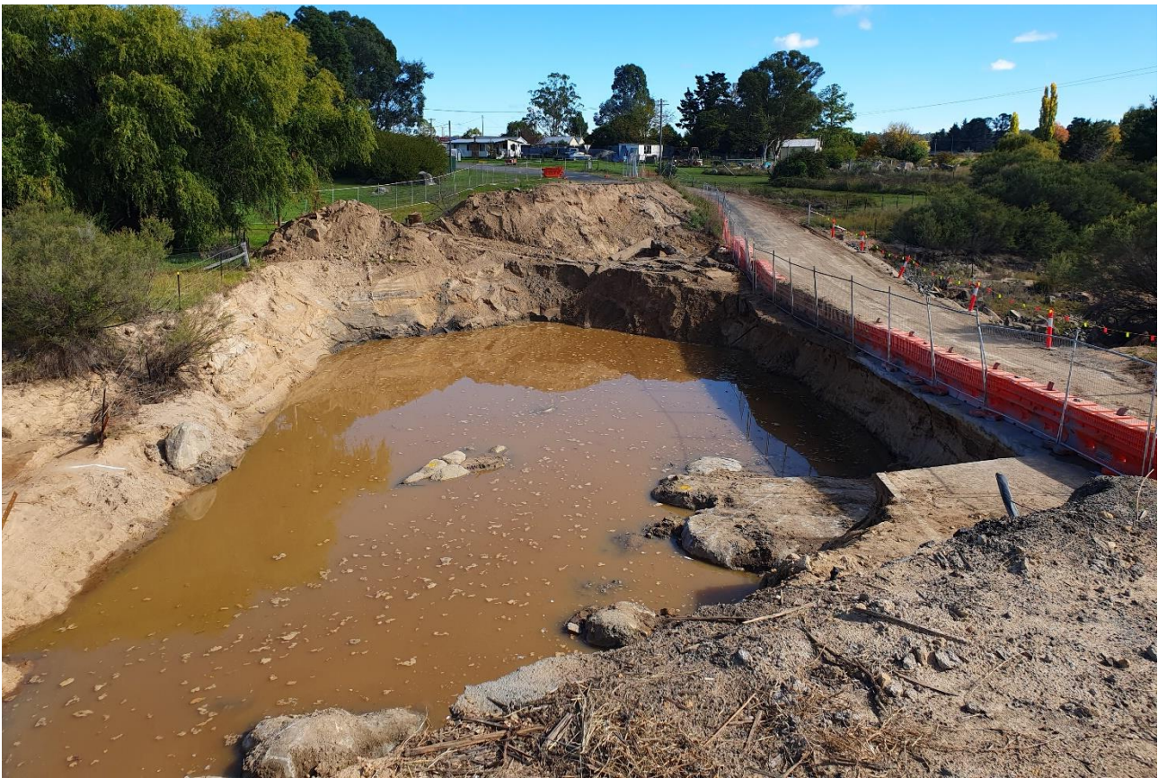
Walkers Bridge Demolition – commencement of foundation excavation
