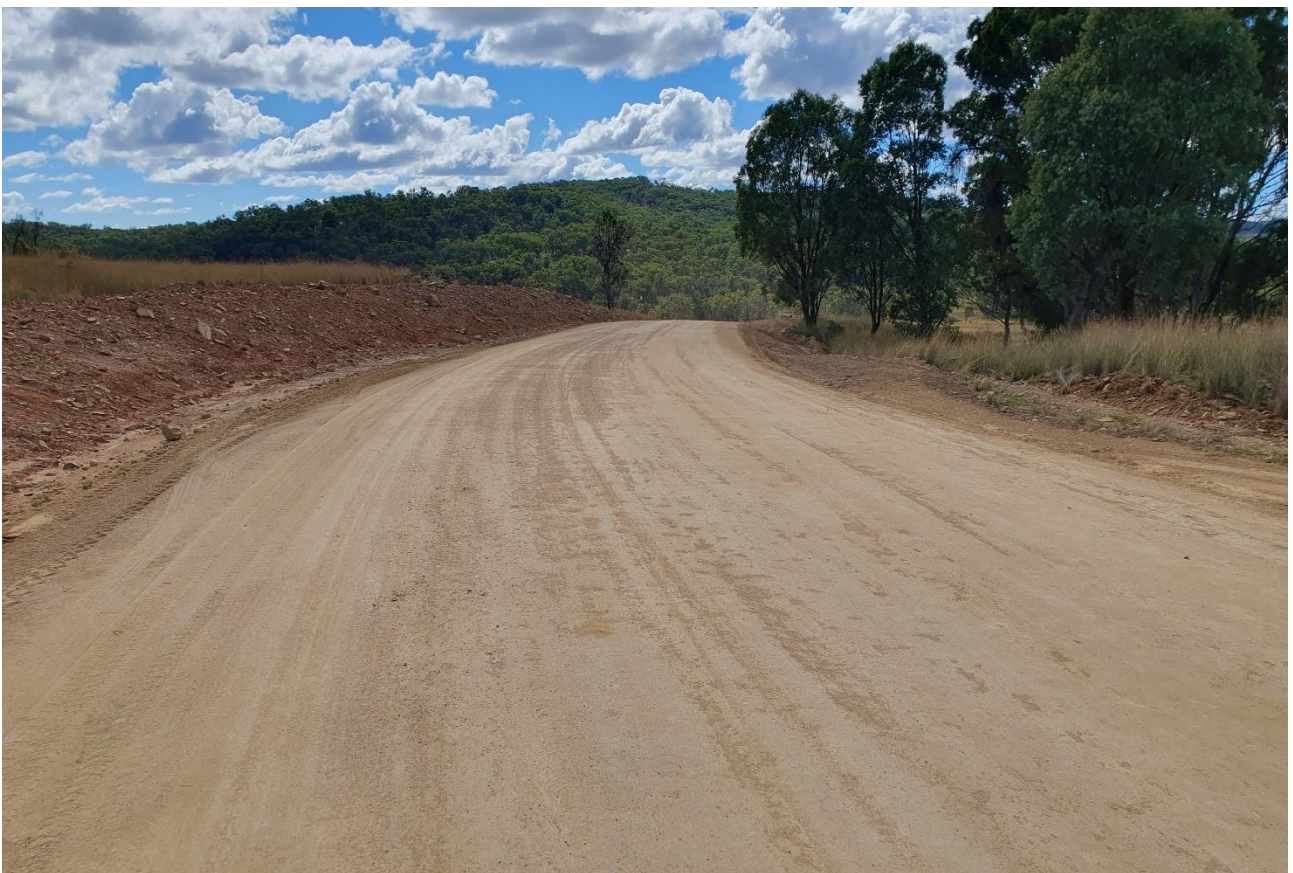
Jones Road Upgrade Project – Earthworks for New Road Formation Completed.
