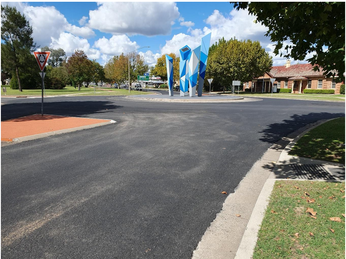
Finished surface Henderson Street Roundabout
