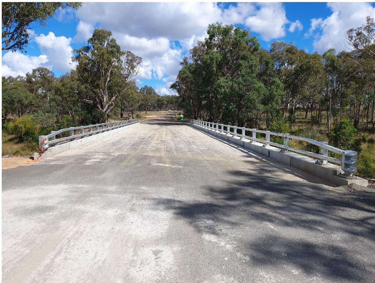
Mathers Bridge – Pavement works completed for the bridge approaches.
