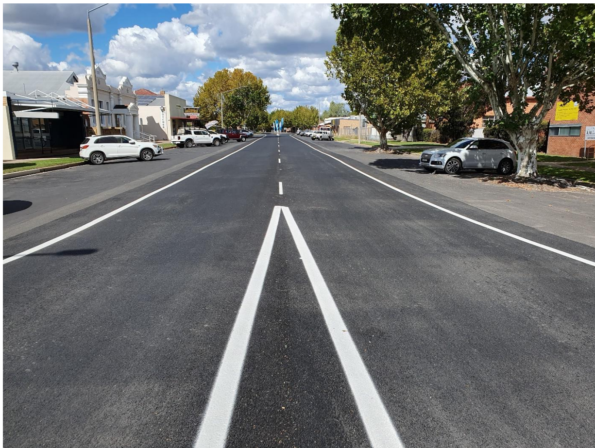
Finished surface Otho Street
