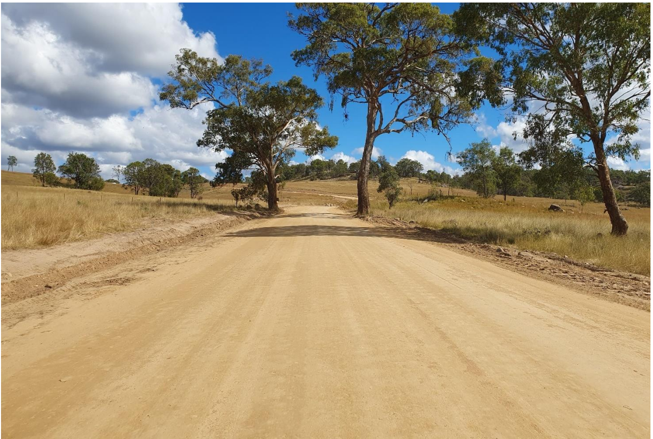
Jones Road Upgrade Project – First Layer of Stabilised Pavement.
