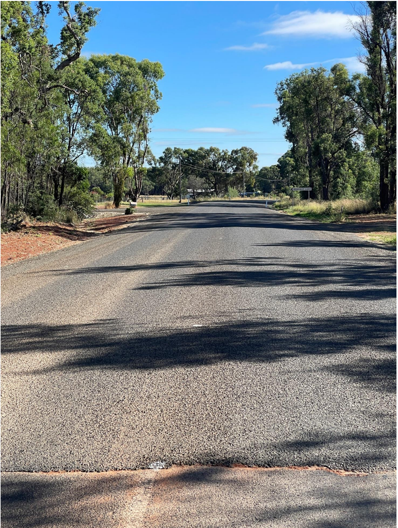
Completed Primer Seal - Intersection of Bonvale Lane.
