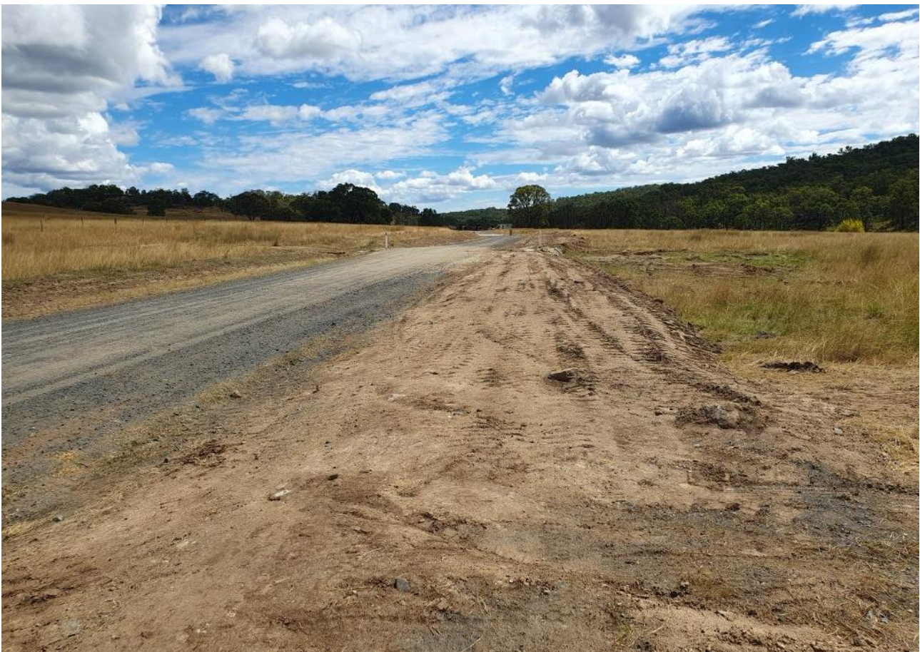
Jones Road Upgrade Project – Earthworks for New Road Formation.
