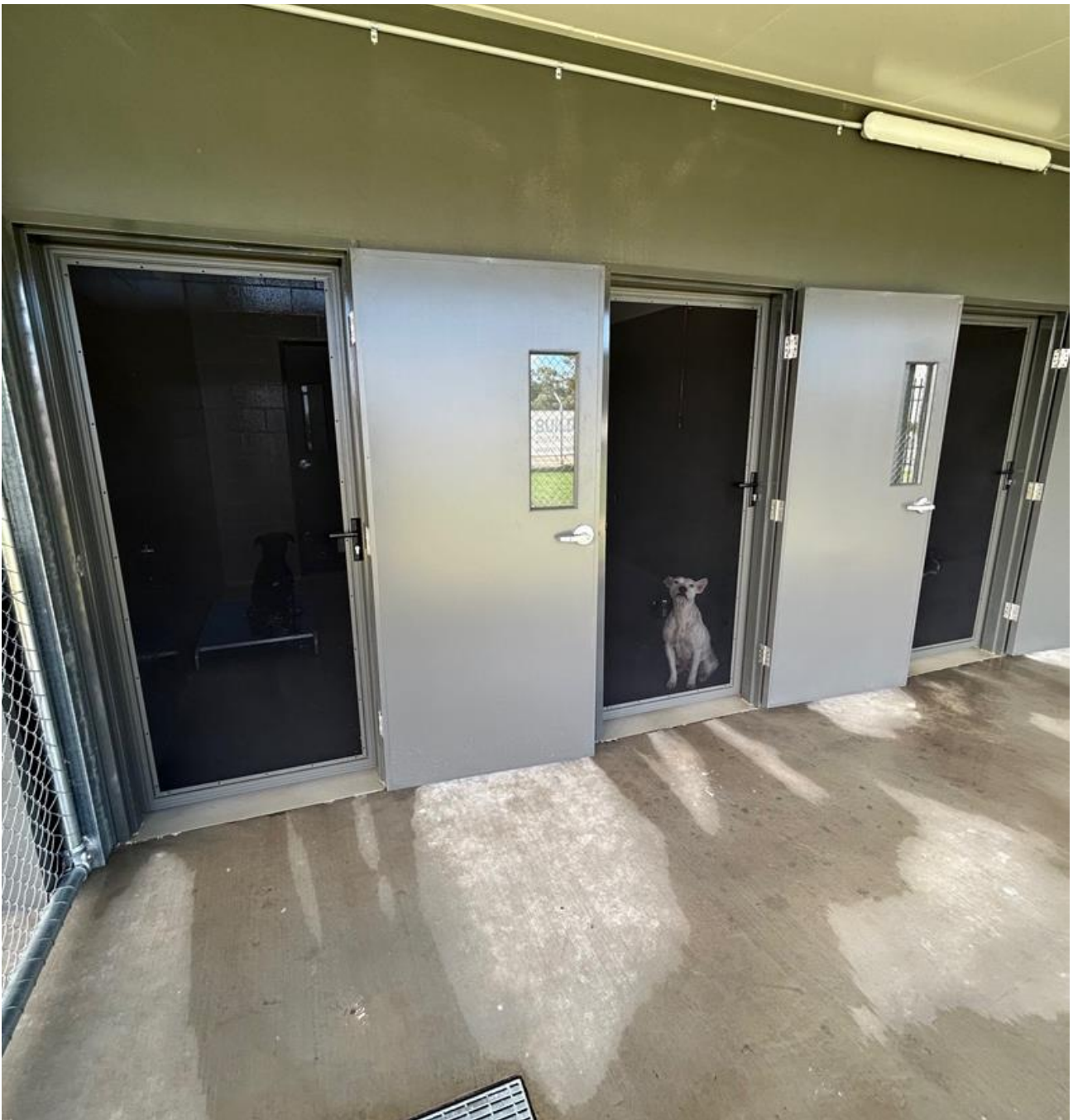
Photo 4- Completed area outside dog holding cells.
