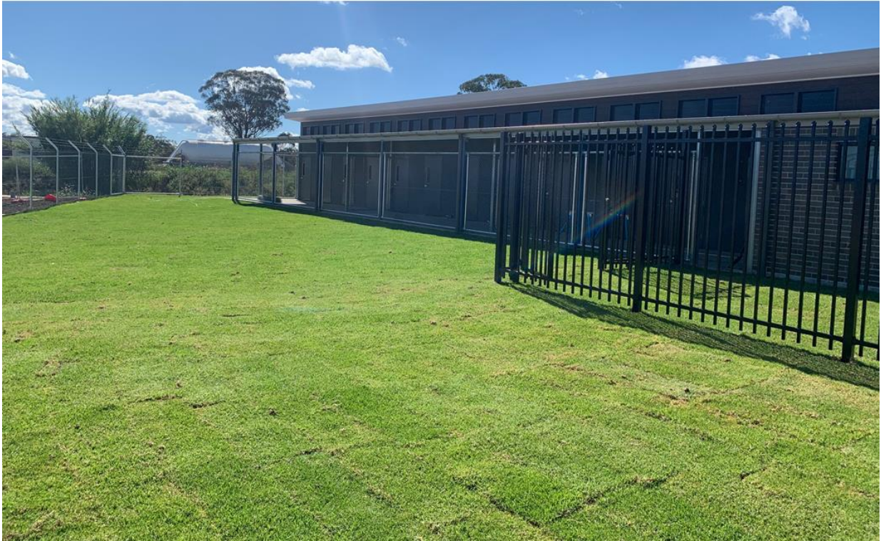
Photo 2: Completed exercise area.
