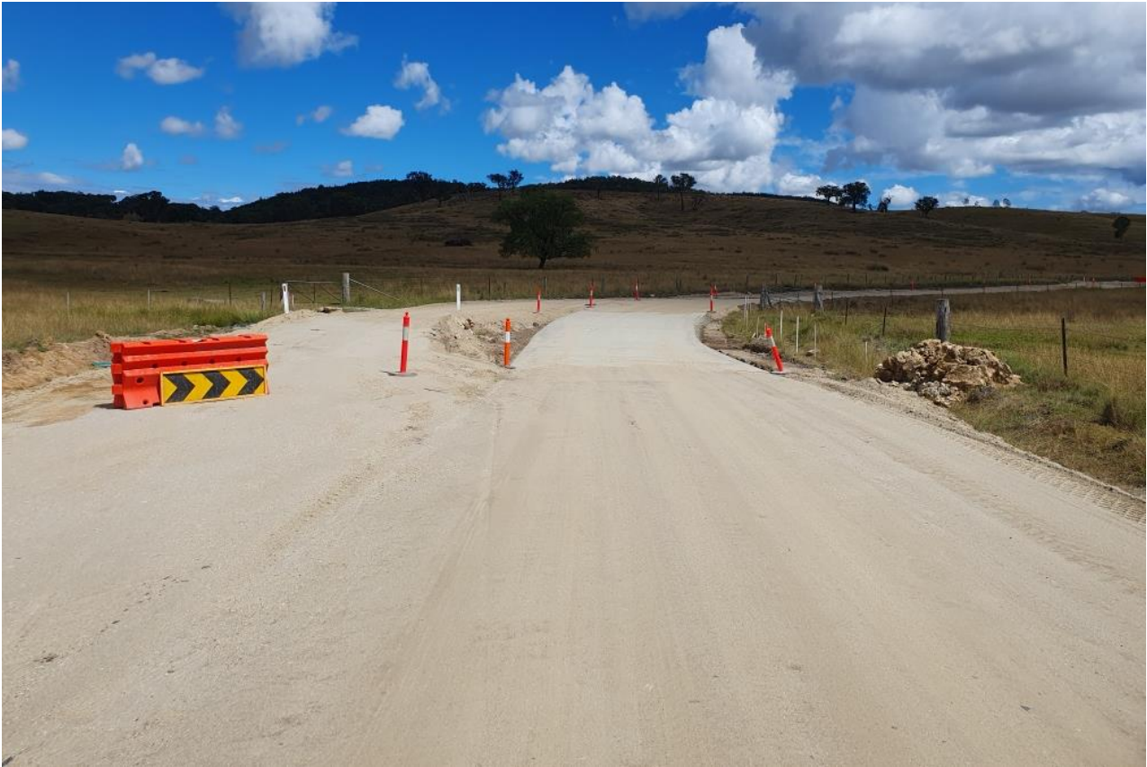
Jones Road Upgrade Project – New Causeway Open to Traffic.
