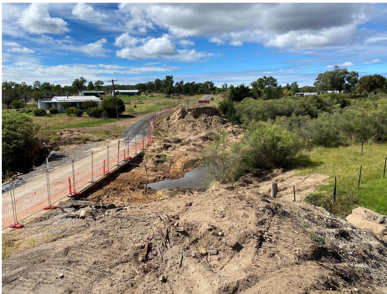
Walkers Bridge Demolition – Removal of Existing Bridge
