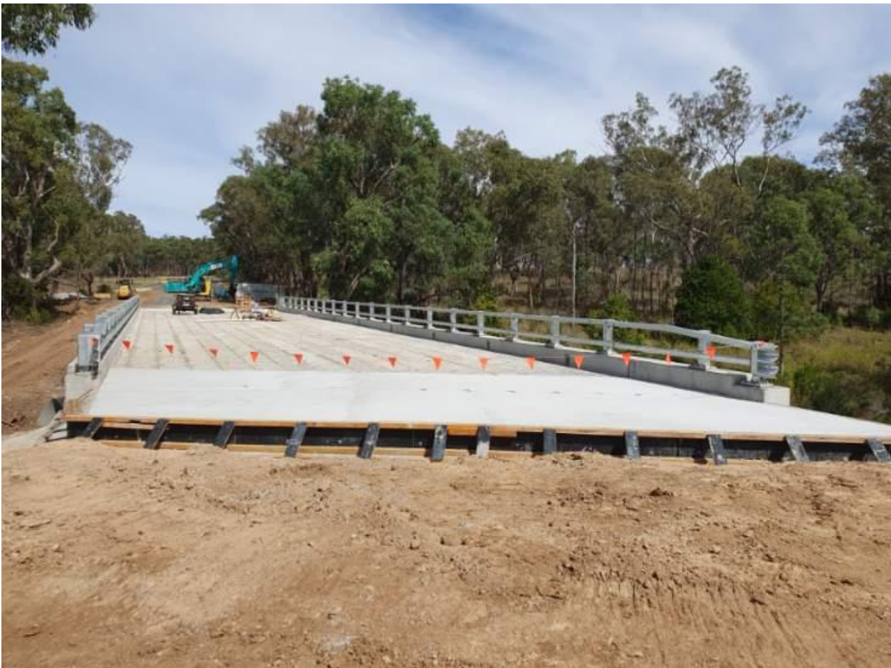
Mathers Bridge – Guardrail and Approach Slabs Installed
