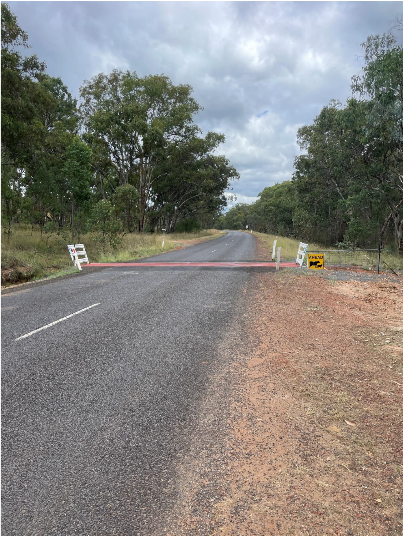
Guyra Road East of Tingha – Installation of Precast Grid.
