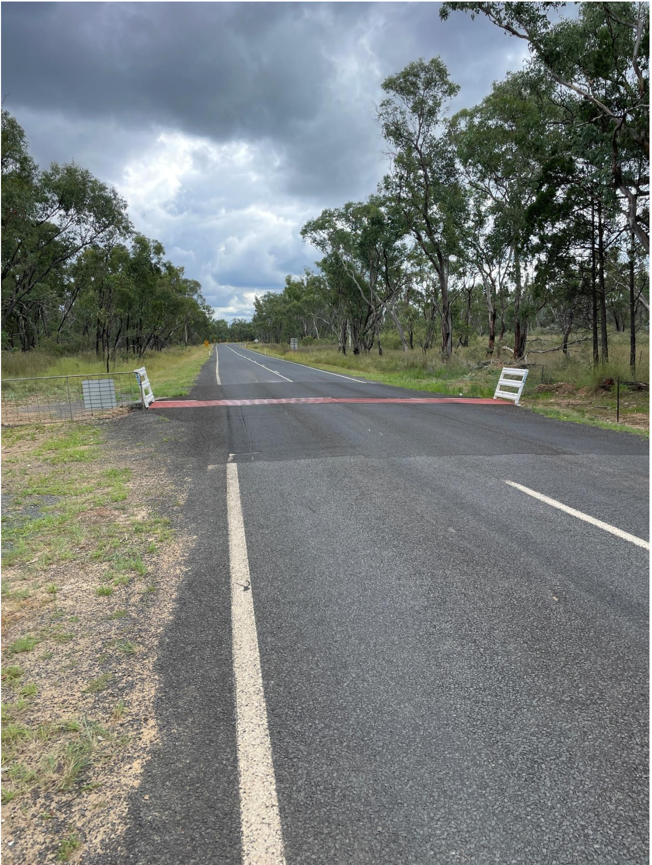
Guyra Road West of Tingha – Installation of Precast Grid.
