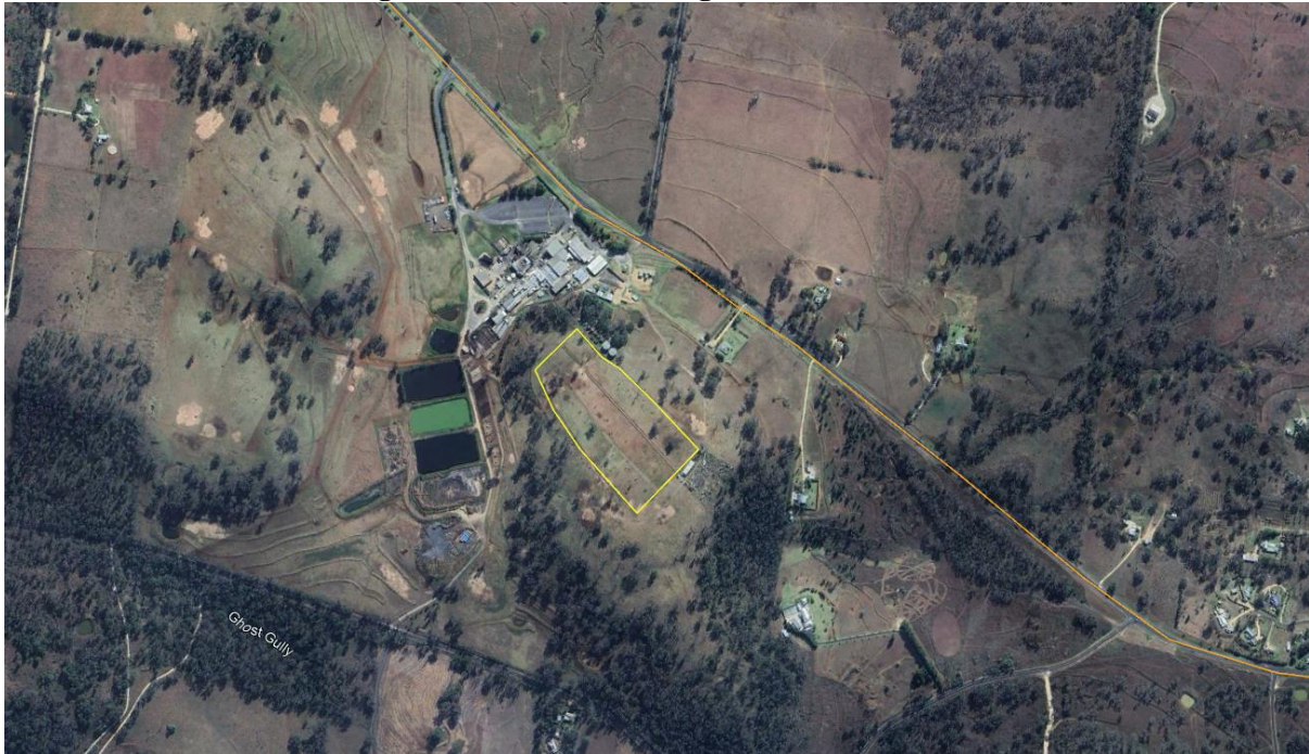
Figure 3: 2023 Aerial image of solar farm site
