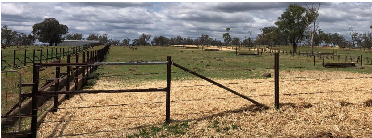
Figure 1: Photo showing ground cover within the cattle yards to be used for the Solar Farm.
