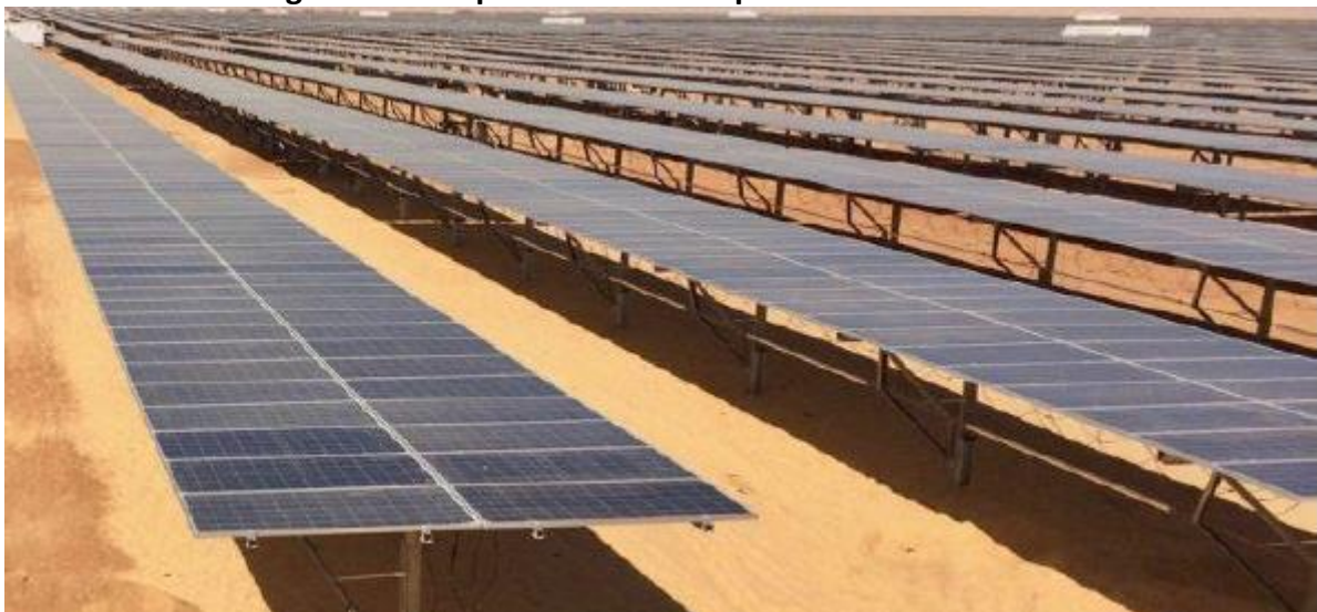
Figure 5: Example of tilted solar panel frame when flat.
