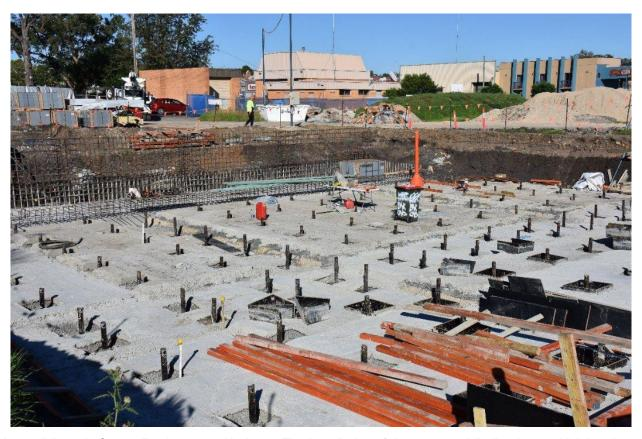
Inverell Aquatic Centre Replacement Update – The installation of the concrete blinding layer which has been installed over the 150mm drainage layer beneath the 50m swimming pool and the extent of the screw piling which has been installed. The screw piling is connected into the structural reinforcement of the concrete pool structure.
