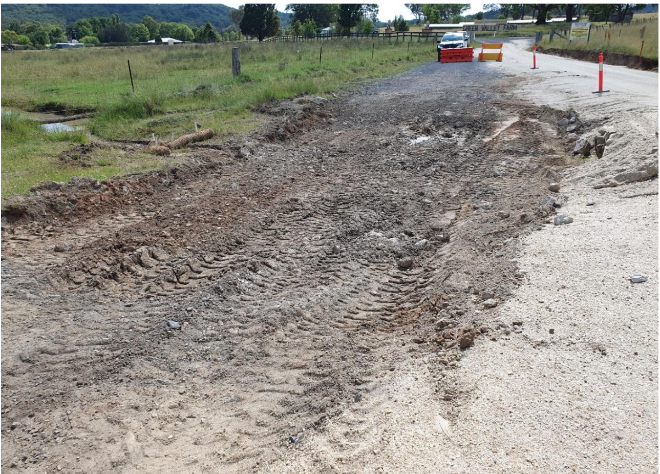
Jones Road Upgrade Project – Existing Causeways have been demolished.
