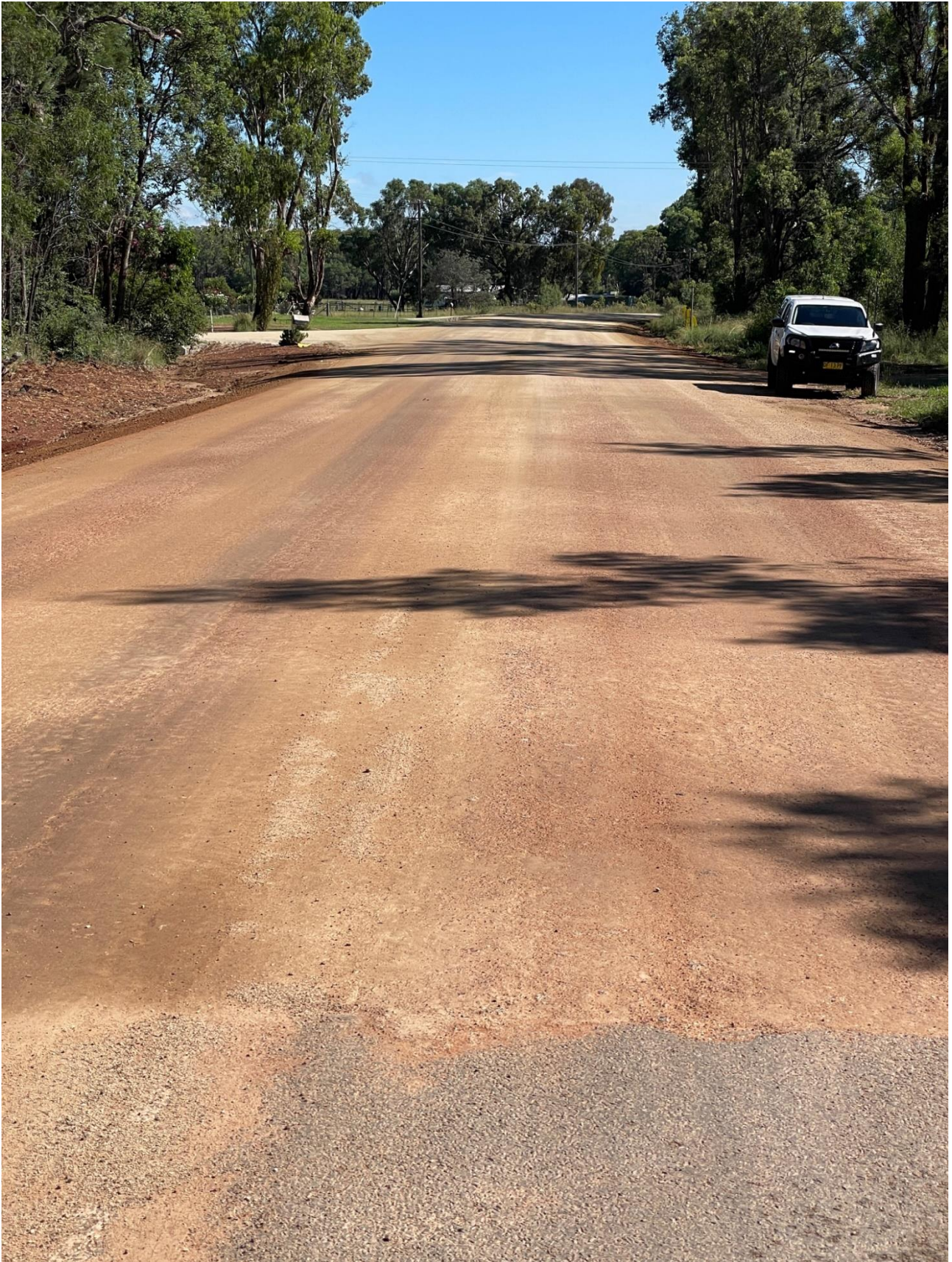
Completed base layer - Intersection Bonvale Lane.
