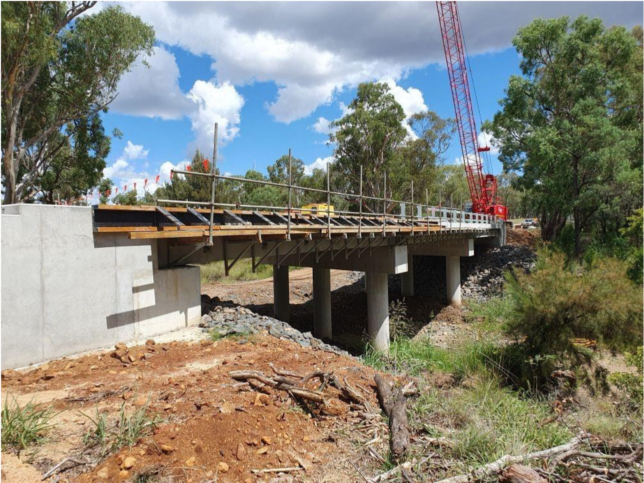
Mathers Bridge – Guardrail Installation
