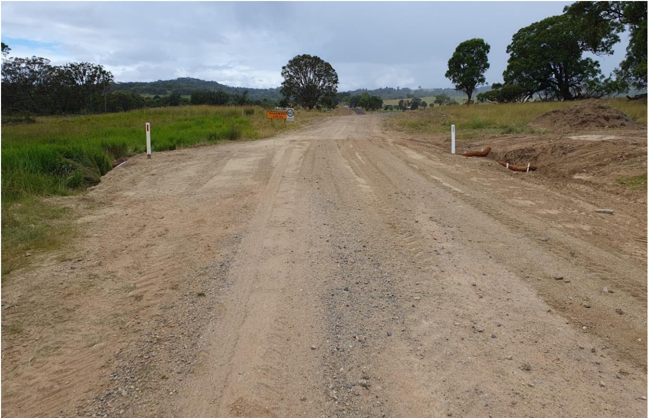
Jones Road Upgrade Project – Drainage pipes installed to suit the new road alignment.
