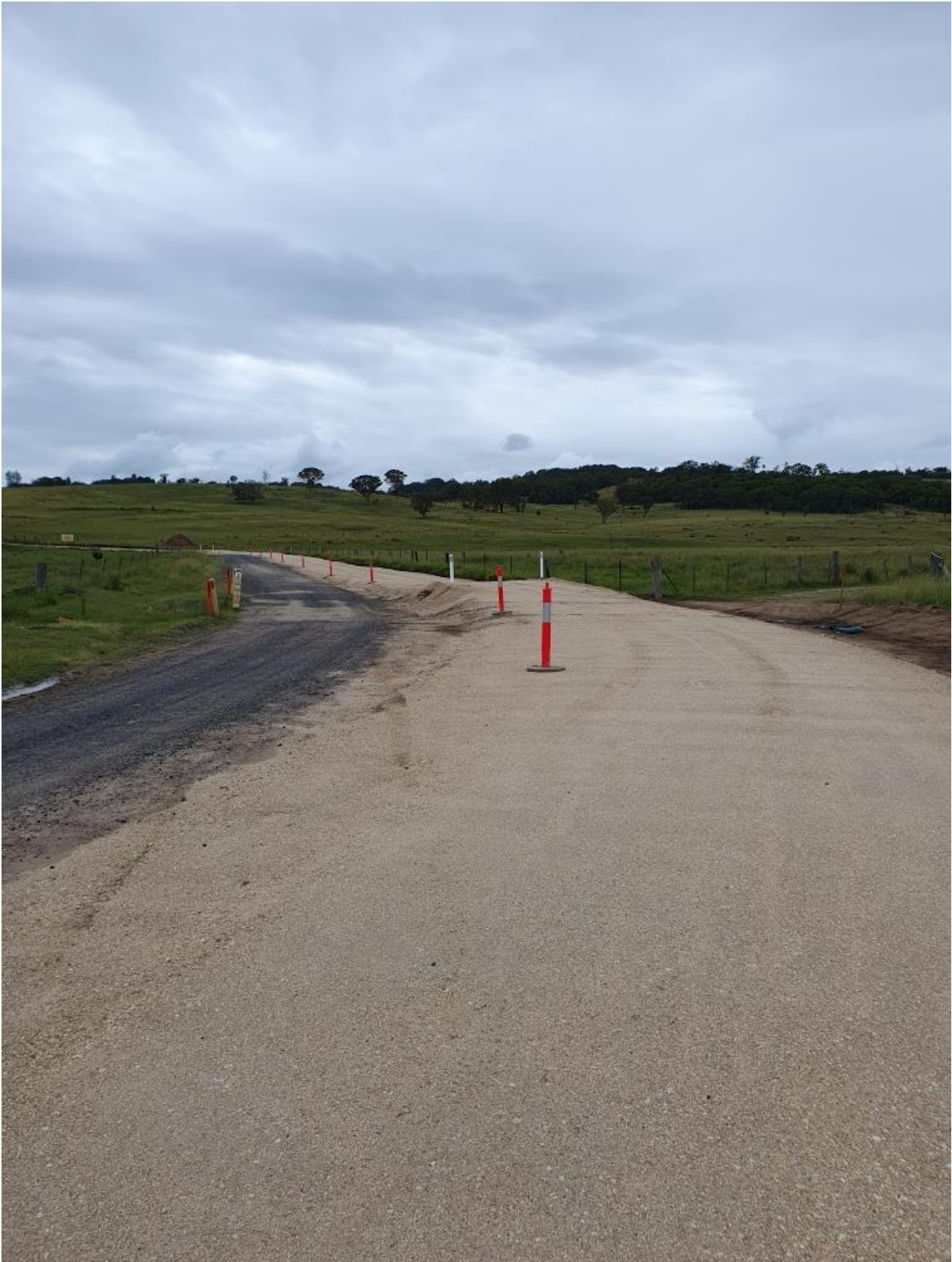
Jones Road Upgrade Project – Side track installed for the replacement of two (2) causeways
