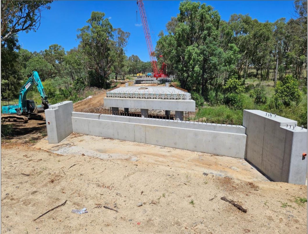
Mathers Bridge Deck Construction underway
