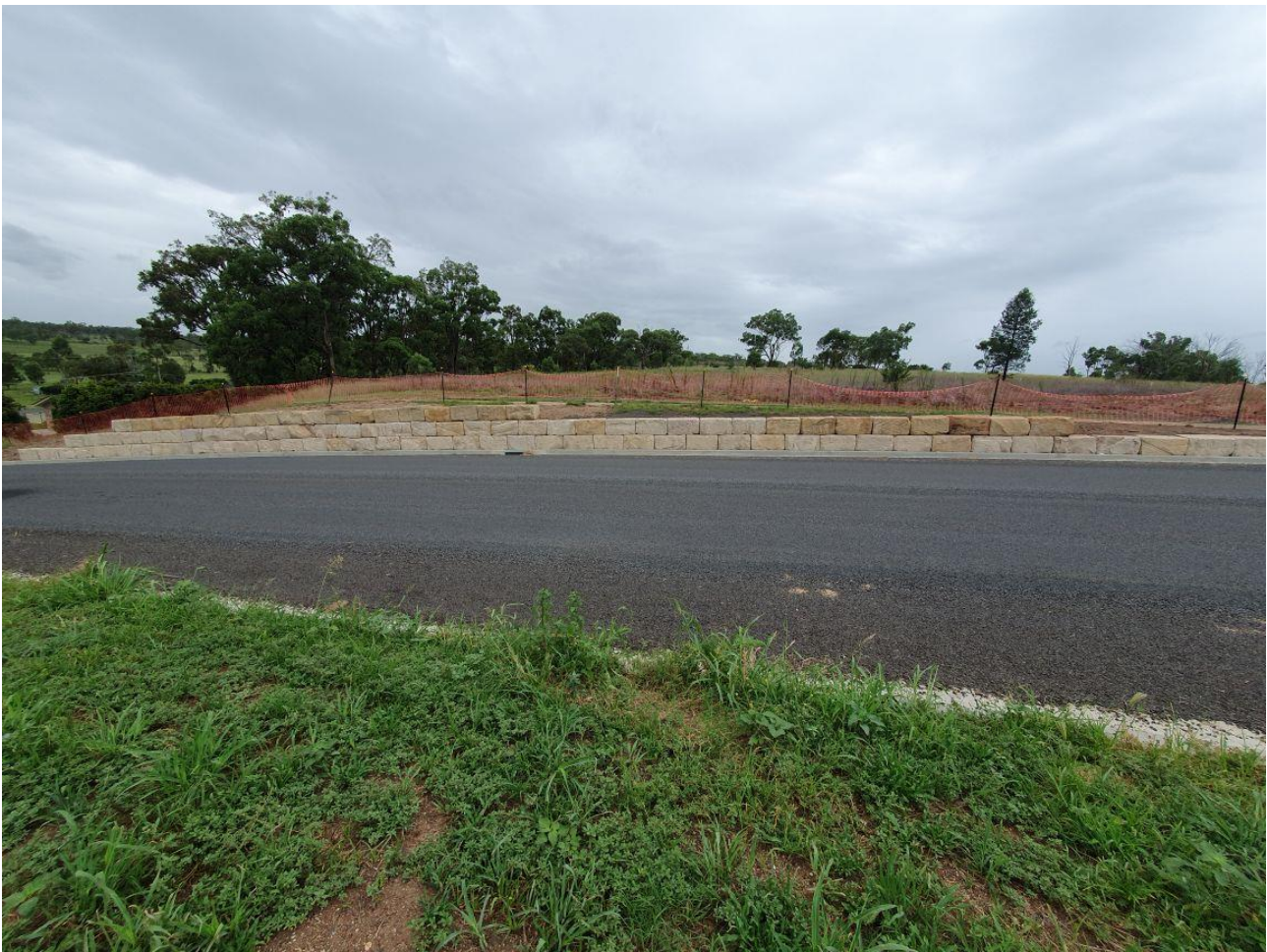
Moore St – Hospital Hill Upgrade – New sandstone block retaining wall on the northern side of the Hospital
