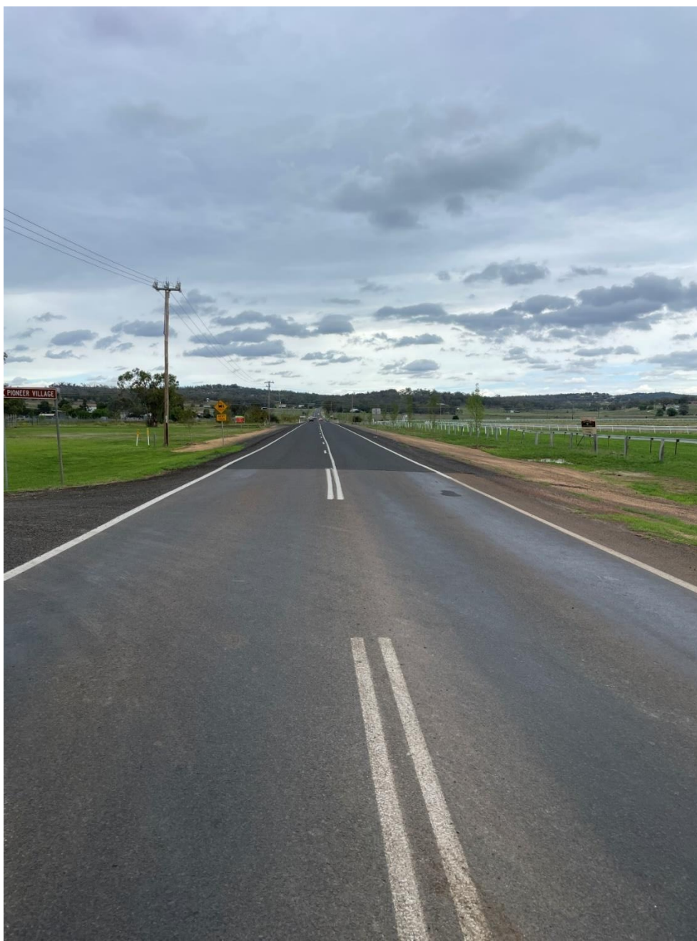
Primer seal and line marking Pioneer Village end
