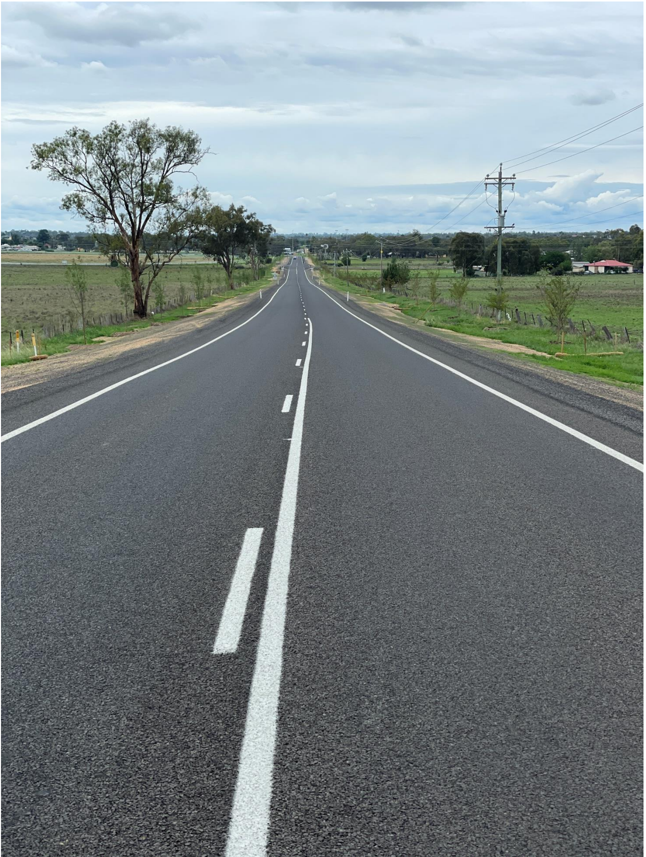
Primer Seal and line marking Cunningham's Hill end Cimmaron Ash on the left side (racecourse side) Crepe Myrtle on the right side
