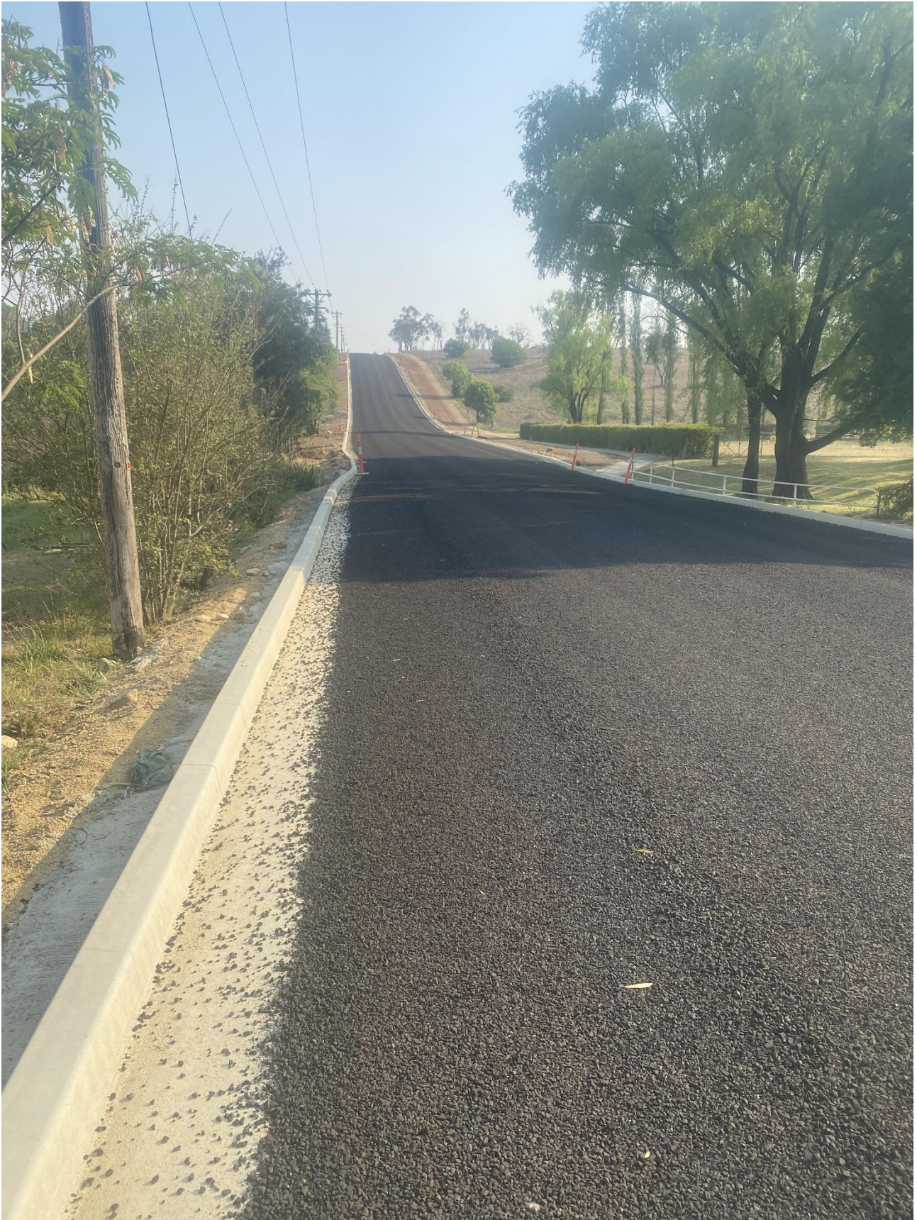
Moore St – Hospital Hill Upgrade – Completed kerb and gutter and sealed southern section
