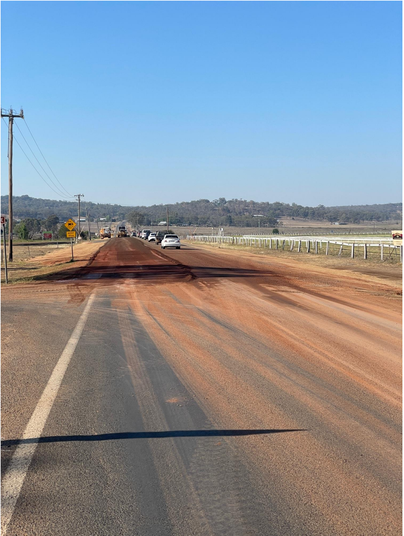
Final trimming of the Base layer in preparation for a primer seal Pioneer Village to Rifle Range Road
