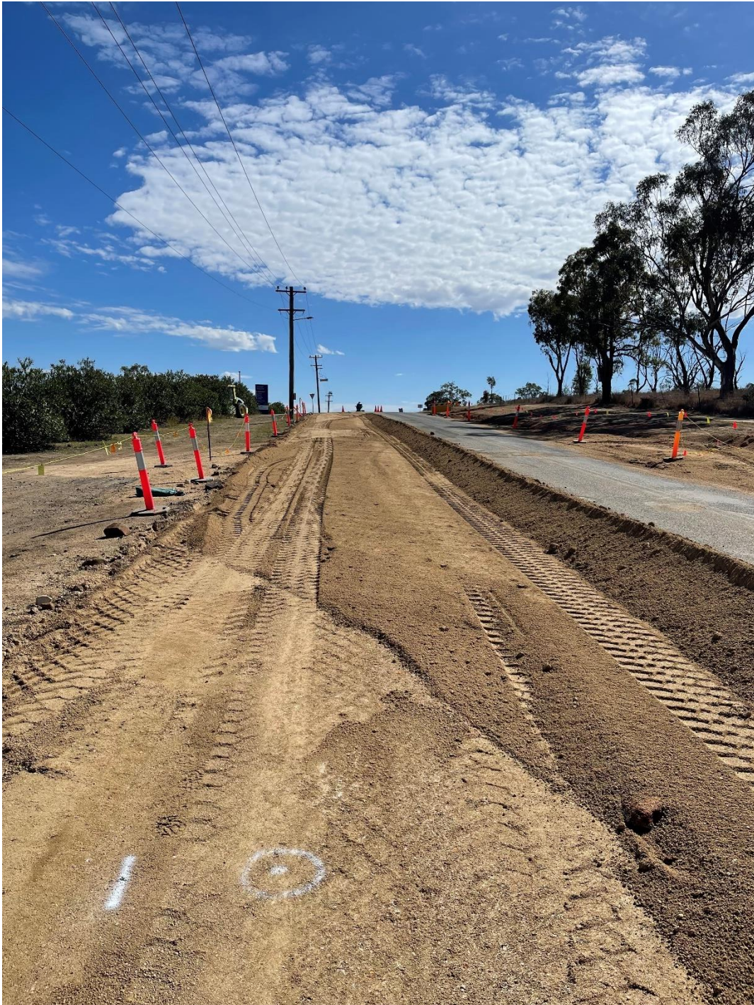
Moore St – Hospital Hill Upgrade – Preparation works for kerb and gutter
