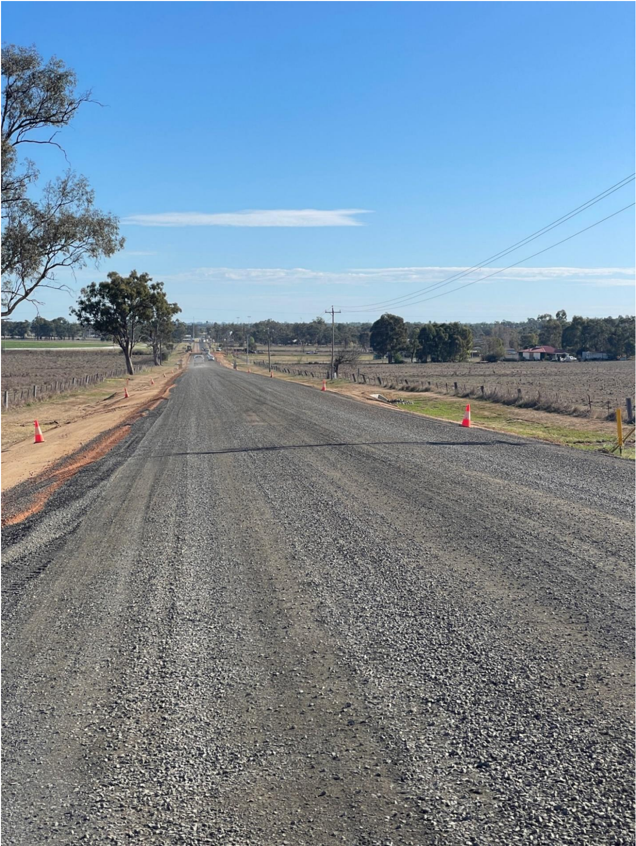
Haulage and spreading of DGB20 Pavement Material for the Base layer
