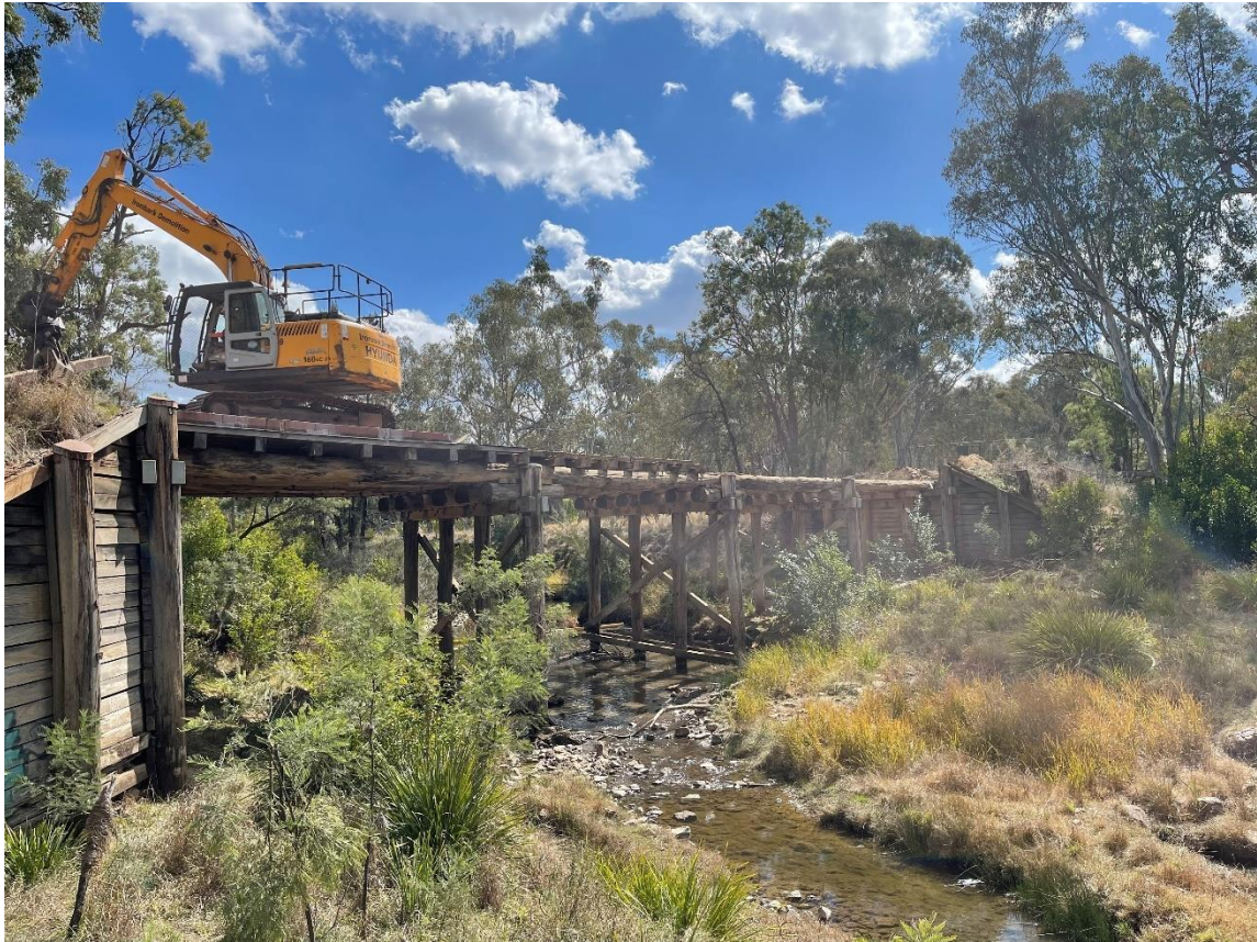
Mathers Bridge Replacement – Demolition of the existing bridge
