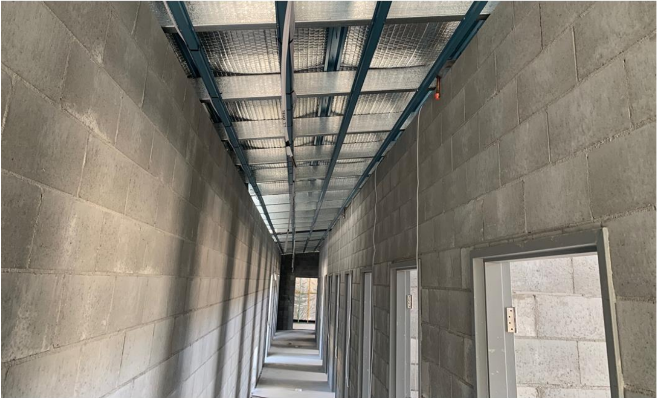
Photo 2 – Ceiling battens and electrical service provisions along hallway.
