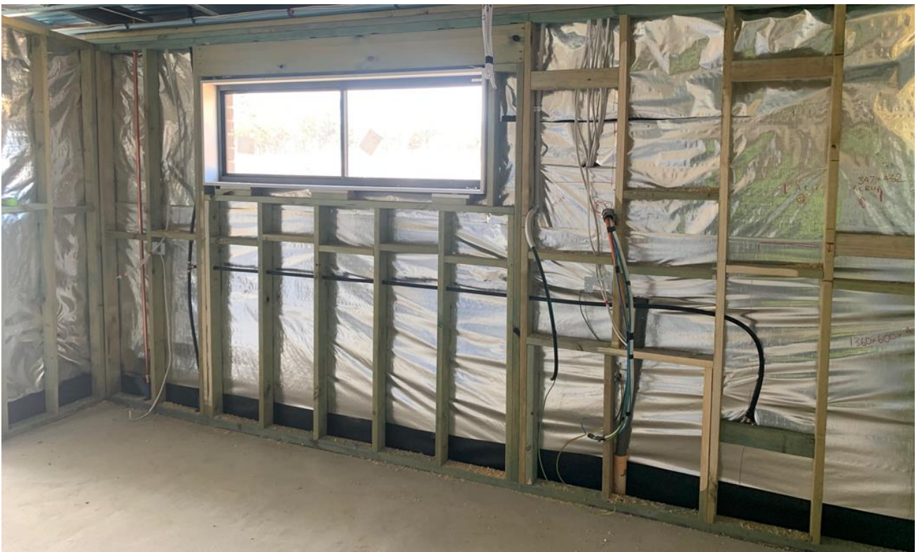
Photo 3 – Installation of plumbing and electrical service provisions in store area of the facility.
