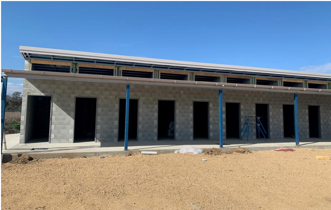
Photo 1- Completed roof members and custom orb roofing.
