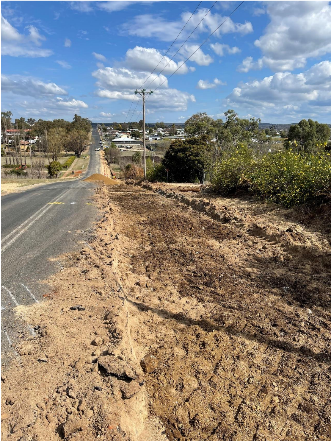
Moore St – Hospital Hill Upgrade – Boxing out of shoulders for kerb and gutter
