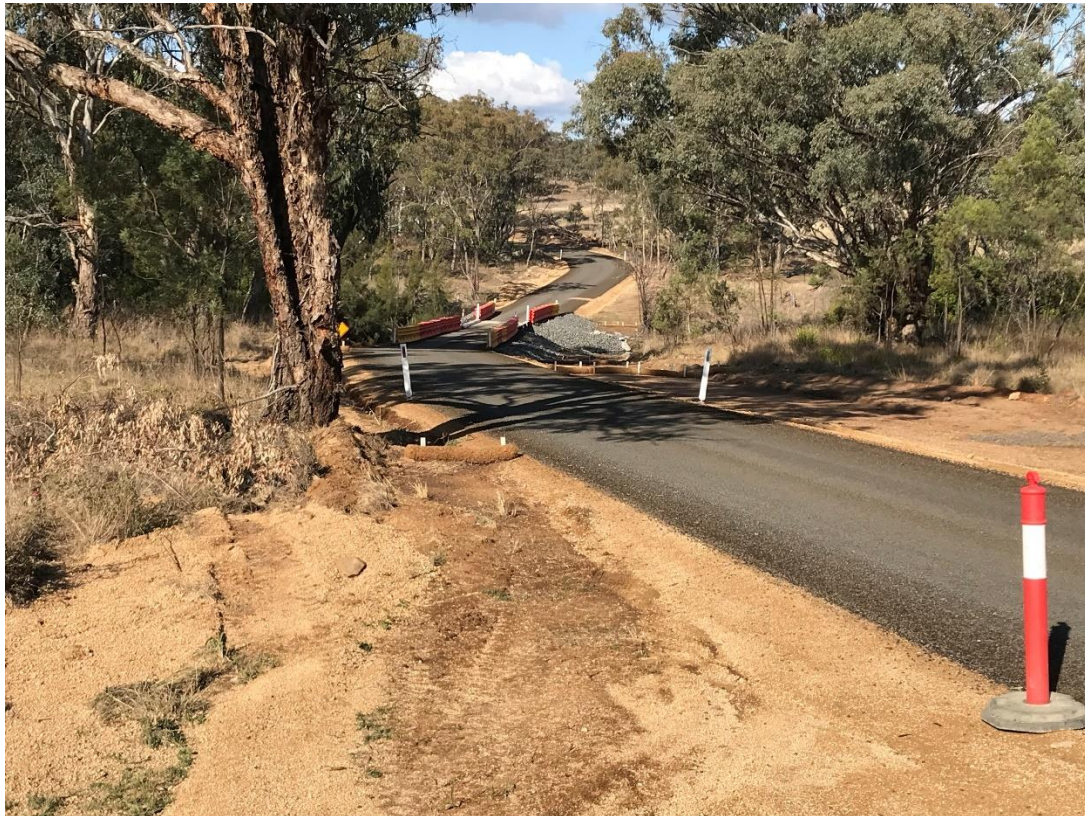
Mathers Bridge Replacement – Temporary Bridge Side Track Open to Traffic
