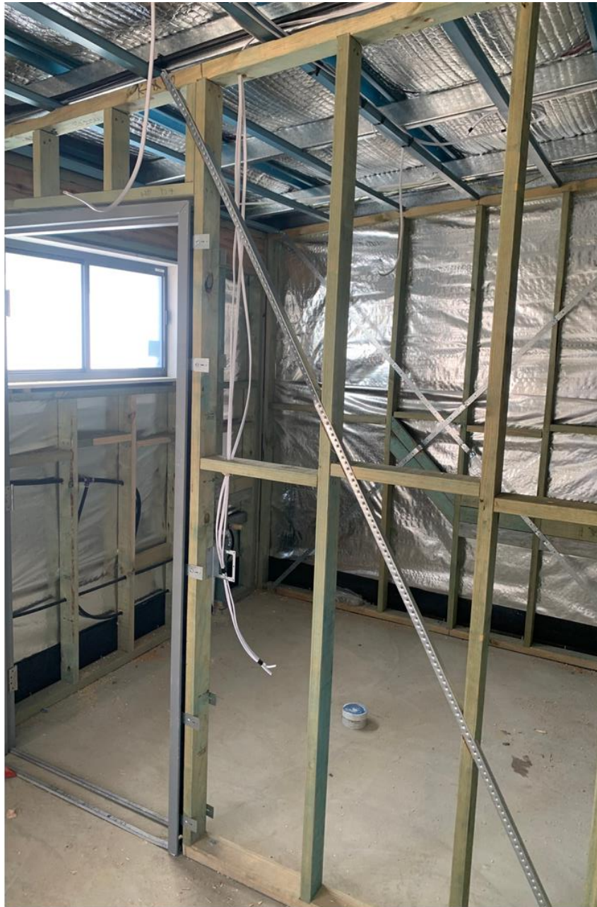
Photo 4 - Completed frame work with plumbing and electrical service provisions installed in accessible amenity area.
