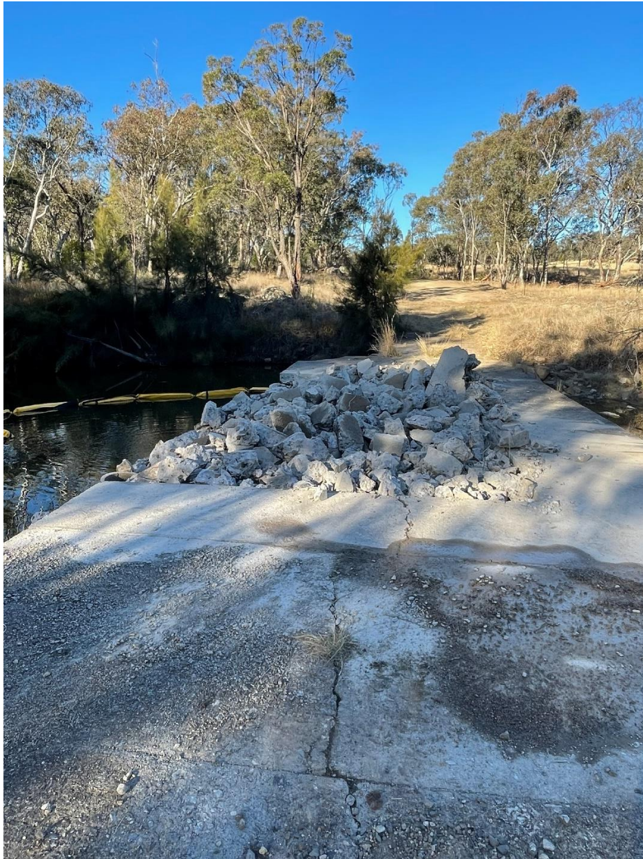
Mathers Bridge Replacement – Existing dilapidated crossing being removed for temporary bridge installation
