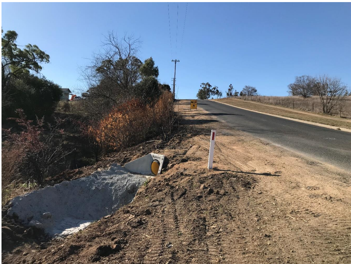
Moore St – Hospital Hill Upgrade – Underground drainage works on the southern side of the hill have been completed
