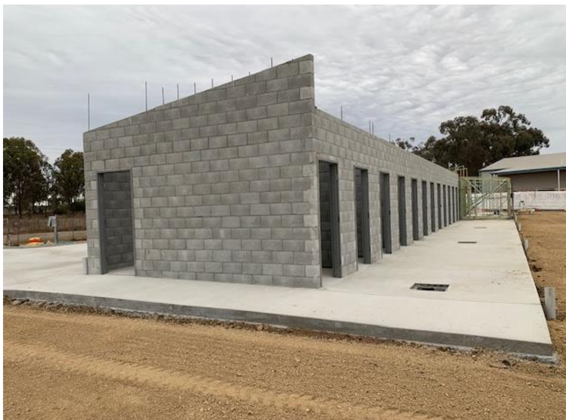
Photo 4 - Completed block work of holding pens.
