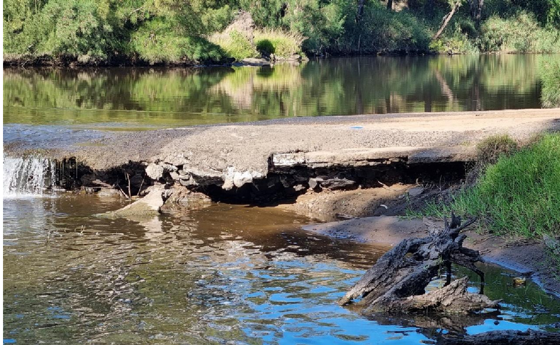
Photograph: Undermining of Holdfast Crossing, 24 March 2023
