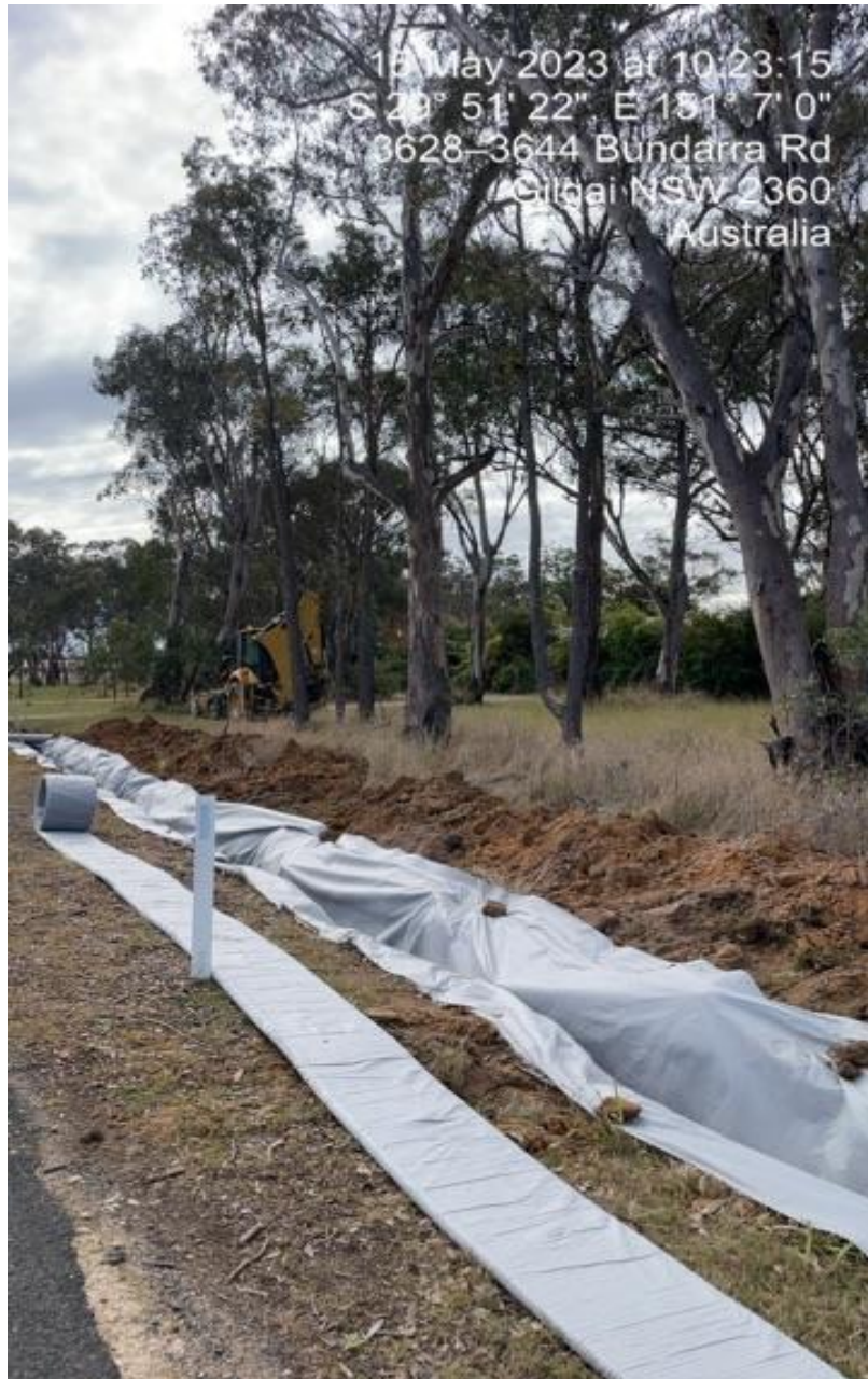
Pro-Drain sub-soil drainage installation
