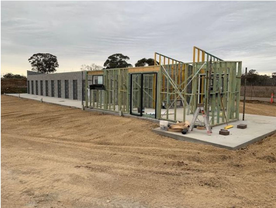
Photo 2 – Timber framework for sanitary facility and reception area.
