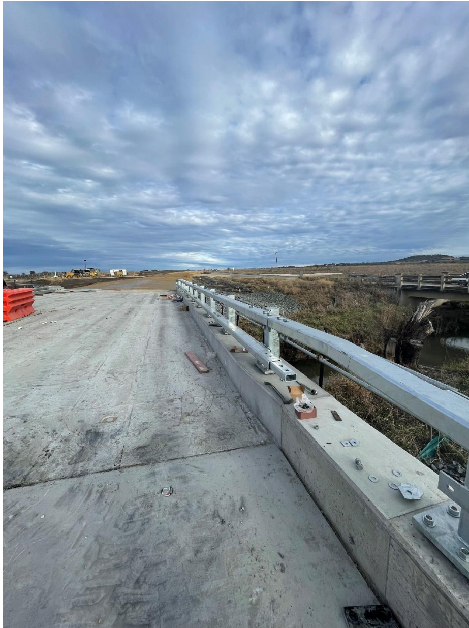
Moseley Dene Bridge Replacement – Guardrail on Bridge
