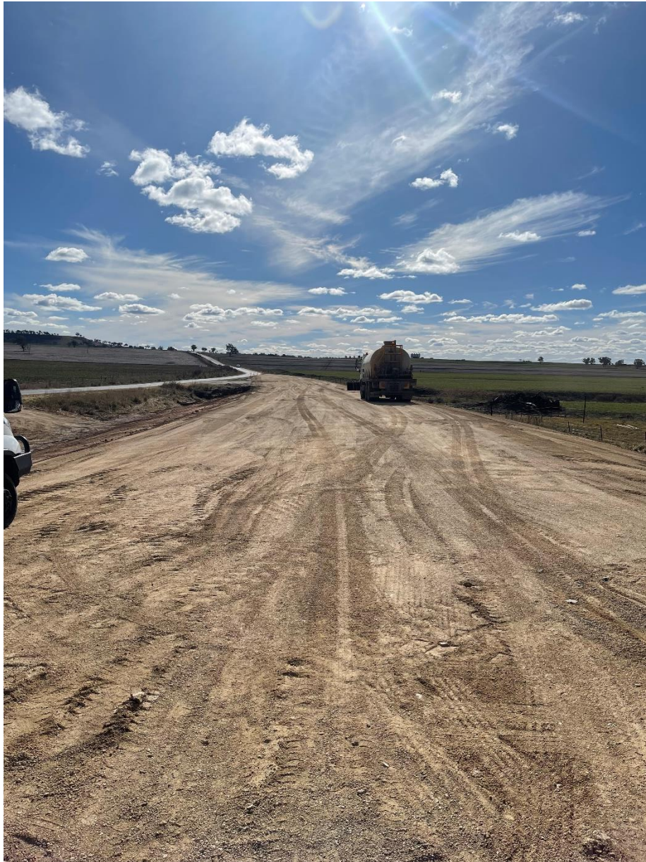
Moseley Dene Bridge Replacement – Road approaches up to finished level awaiting tie-ins
