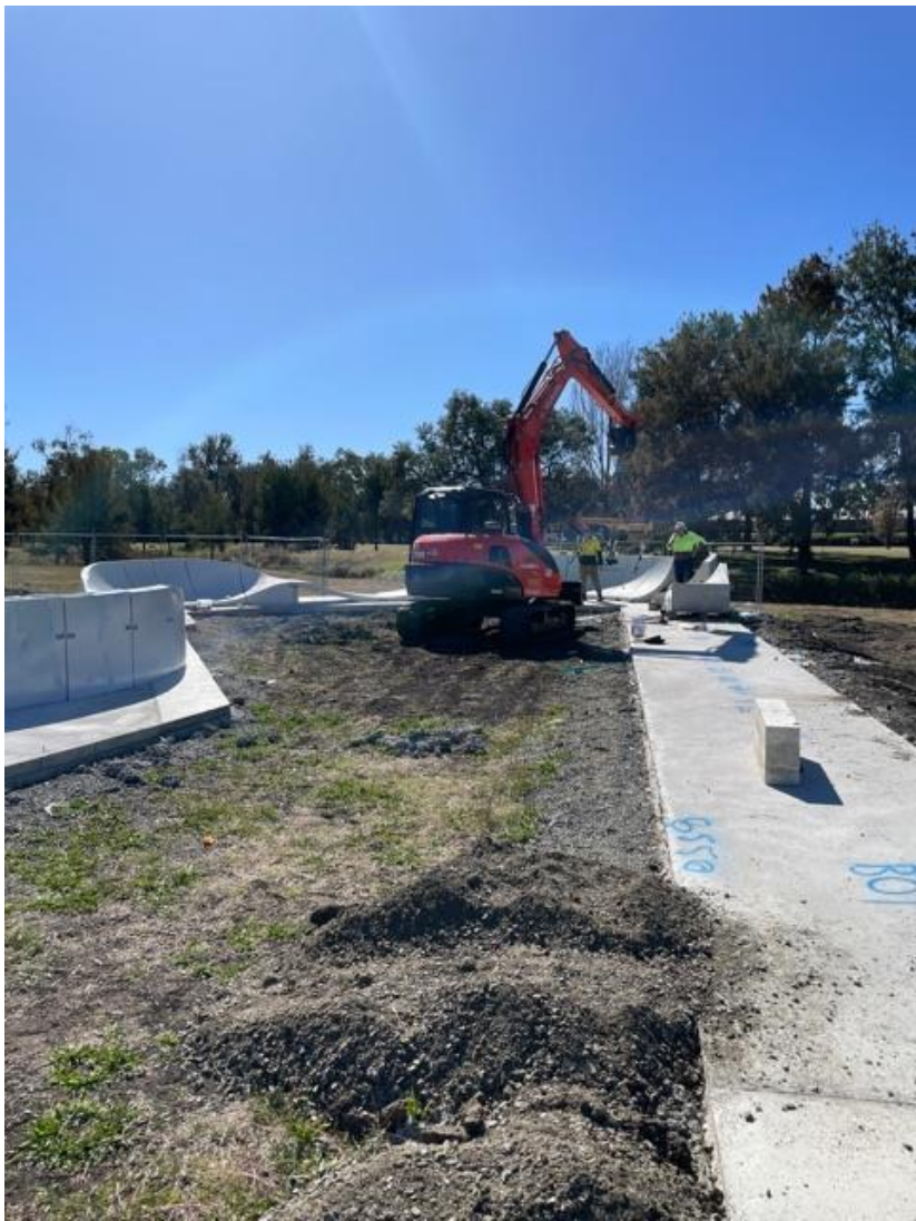
Installation of pump track components
