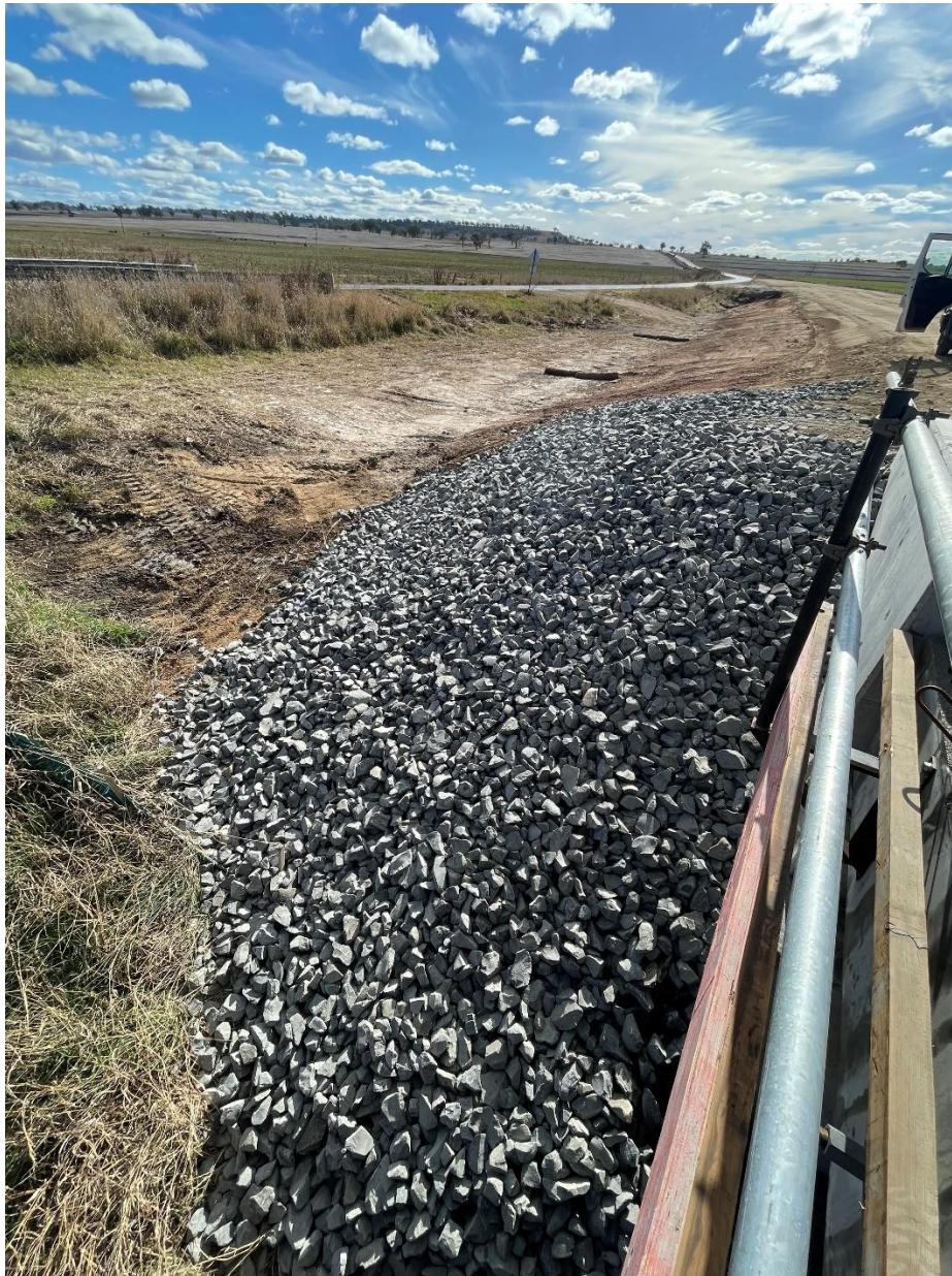
Moseley Dene Bridge Replacement – Rock batter protection in place
