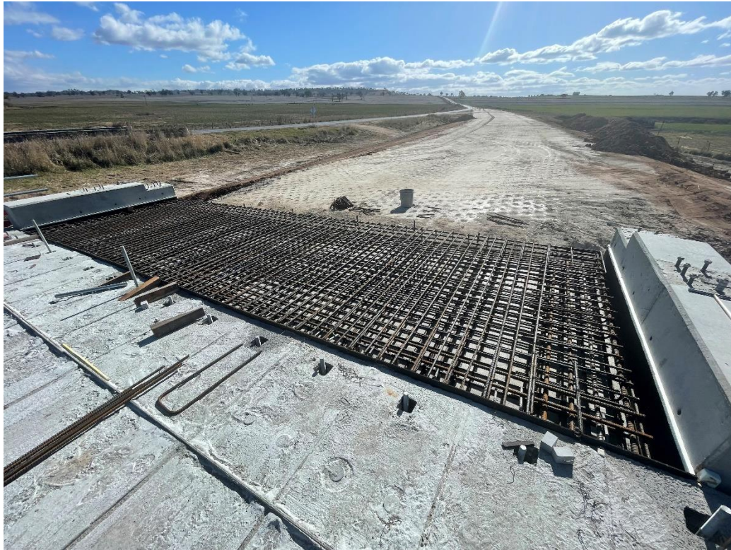
Moseley Dene Bridge Replacement – Relieving Slab Steel Reinforcing
