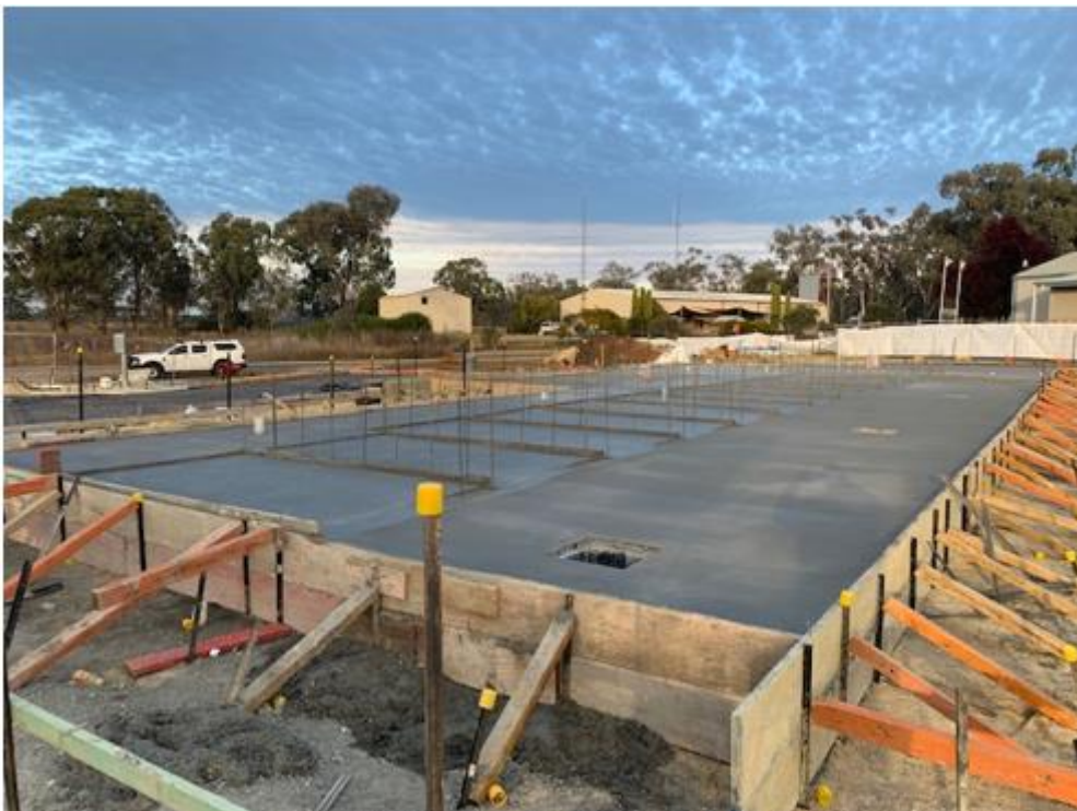
Photo 3 - Concrete slab after concrete placement
