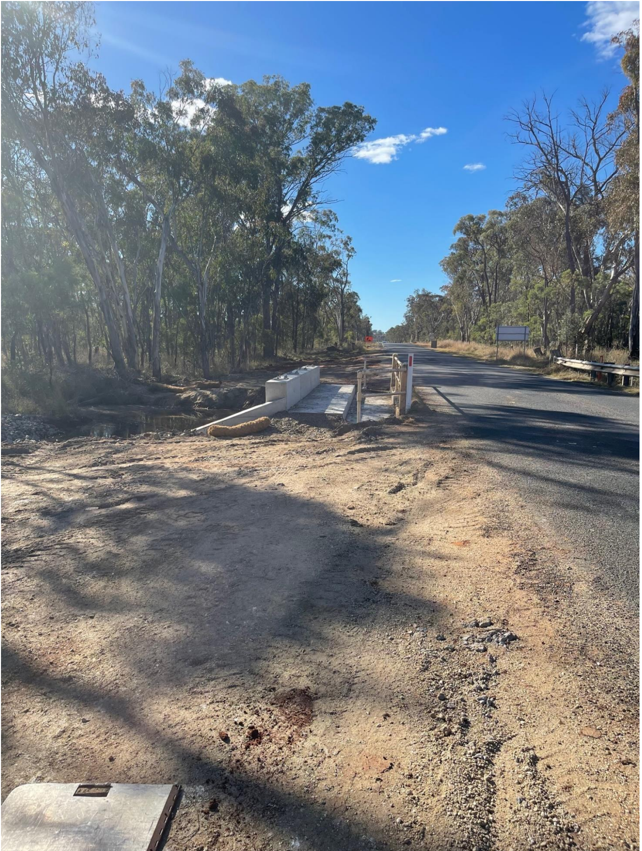
Box culvert extension Gilgai Creek Tributary
