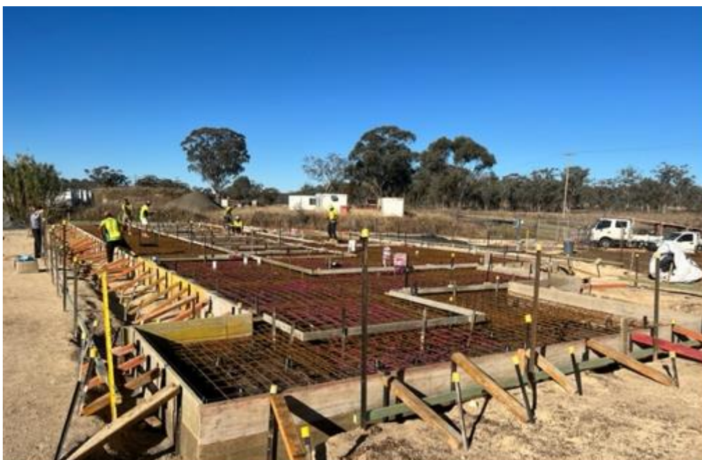
Photo 1 - Preparation of concrete slab formwork and steel reinforcement.
