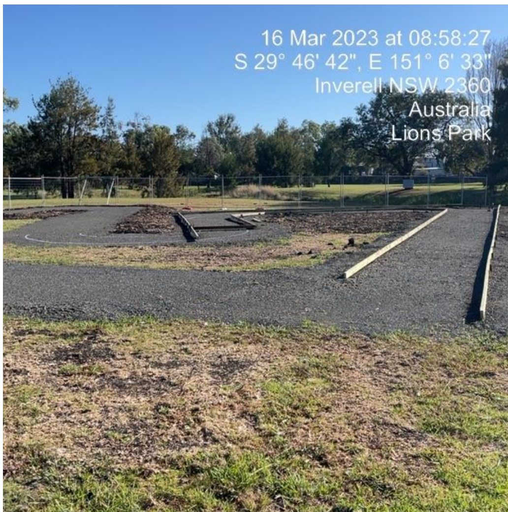
Pump track earthworks and concrete base slab preparation works
