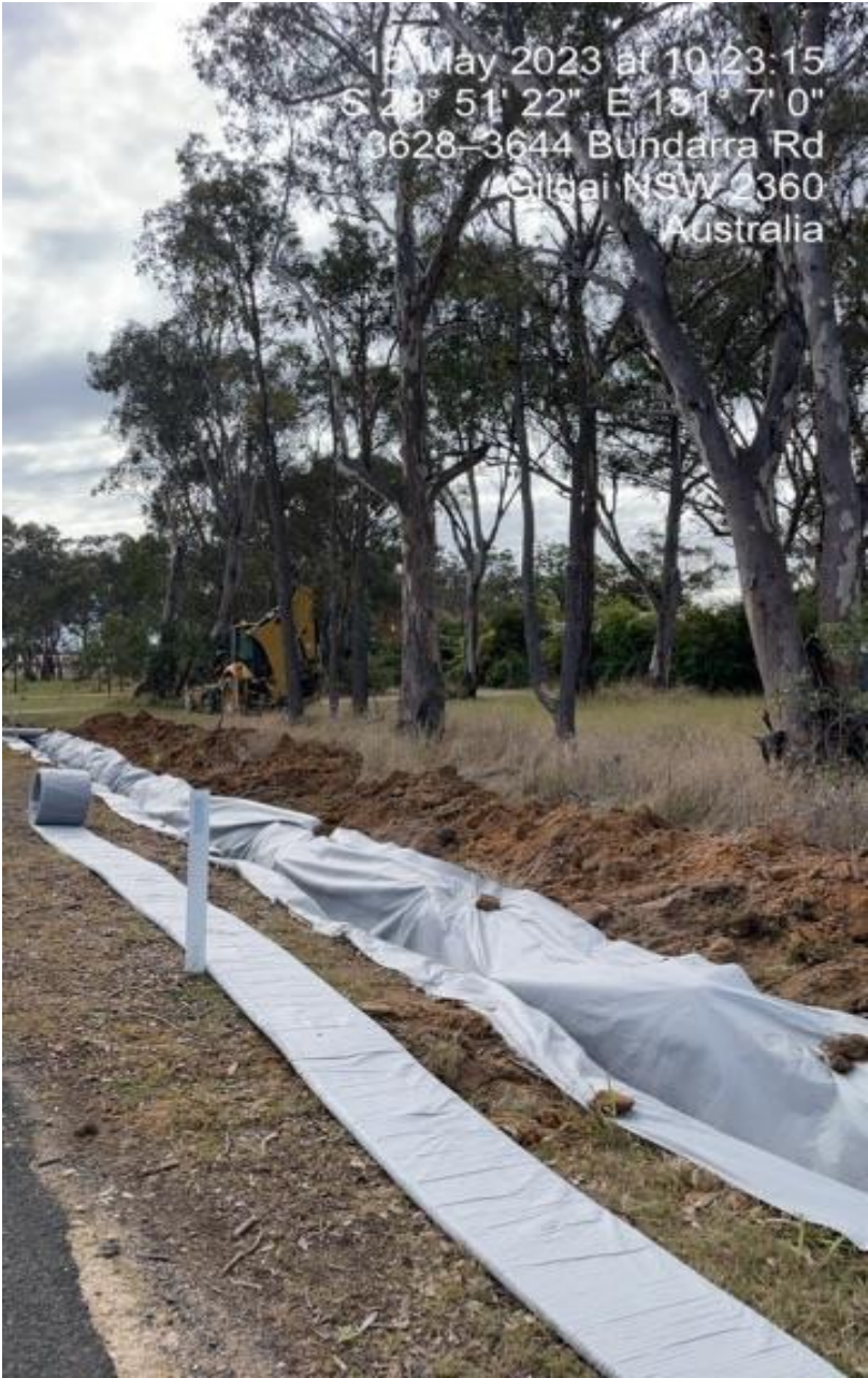
Pro-Drain sub-soil drainage installation
