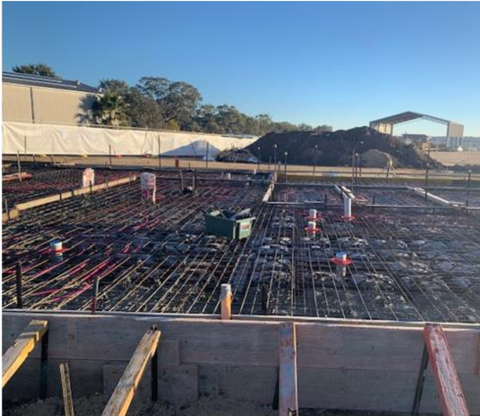
Photo 2 - Concrete slab formwork, reinforcement, drainage penetrations and underfloor heating.
