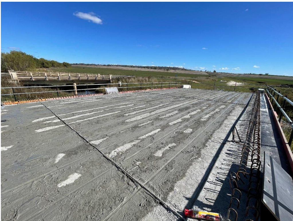
Moseley Dene Bridge Replacement – Bridge decks in place ready for post-tensioning
