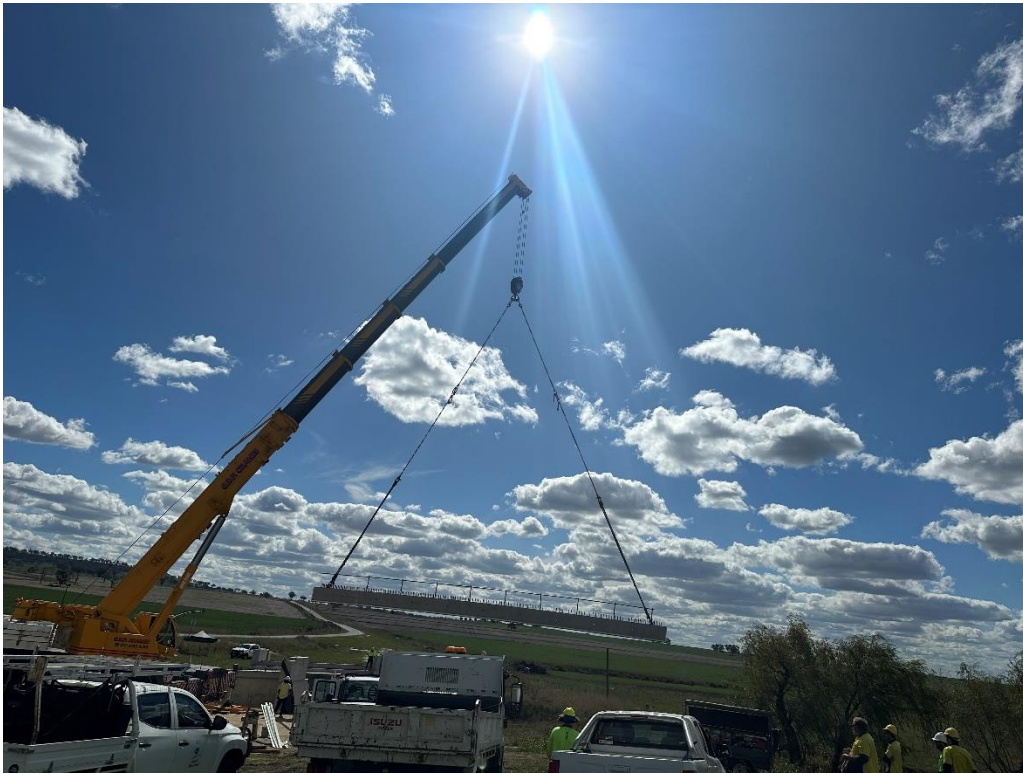
Moseley Dene Bridge Replacement – Lifting bridge planks into place
