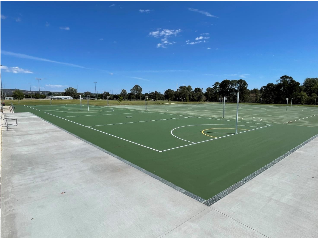
Inverell Netball Court Upgrade – Plexipave Surface and linemarking completed
