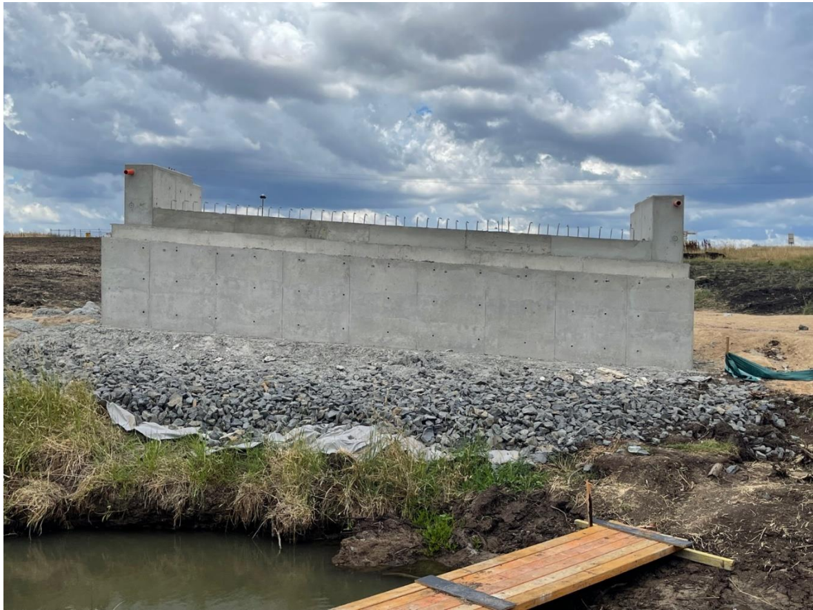
Yetman Road – Moseley Dene Bridge Replacement Project – Abutments and Wingwalls completed
