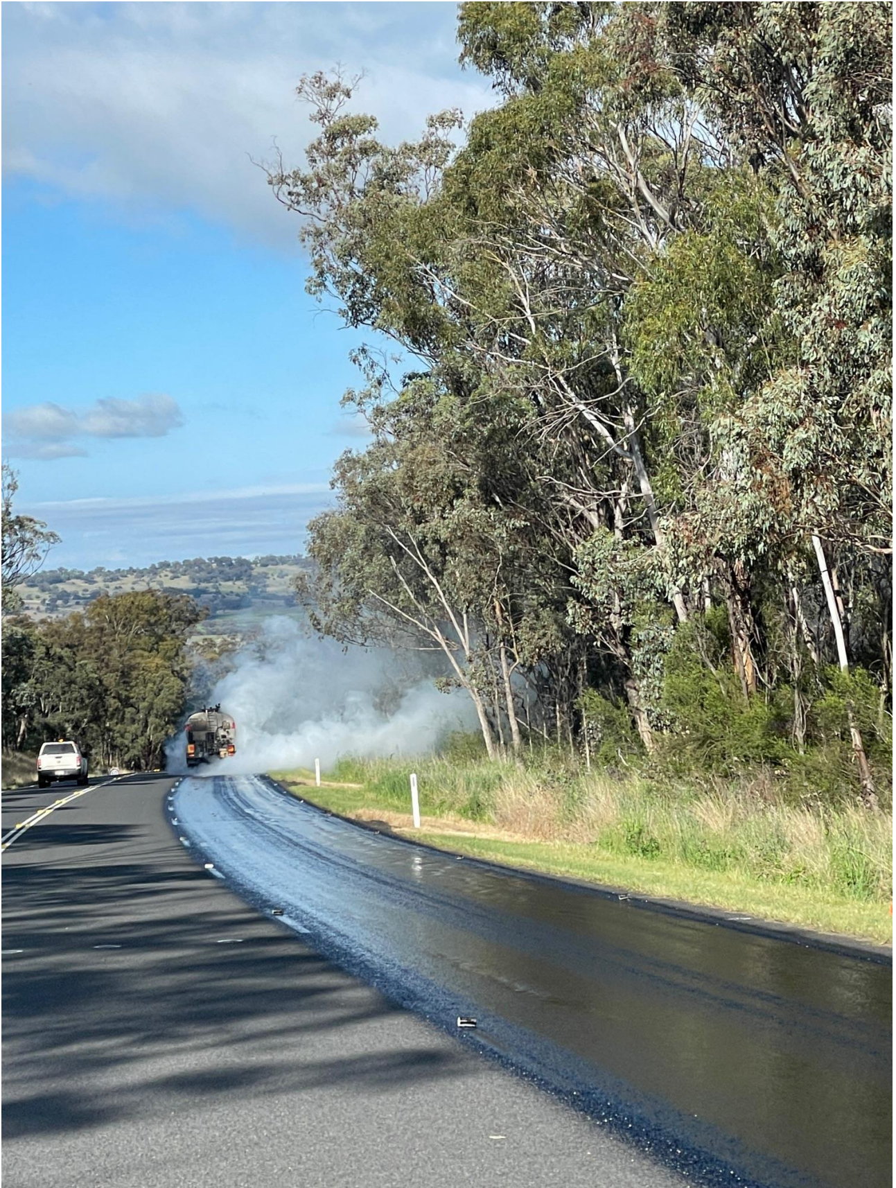
Spraying of Bitumen – Gwydir Highway East of Inverell
