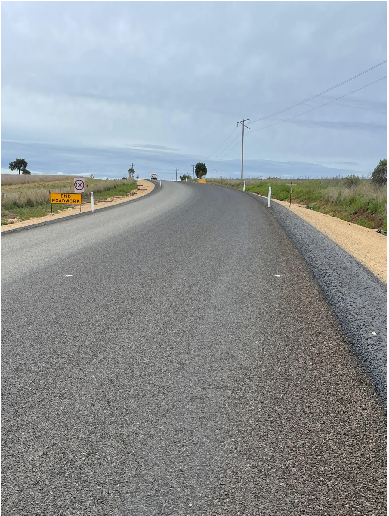
Completion of Primer seal – Ashford Road Wandera South – Northern end of project site
