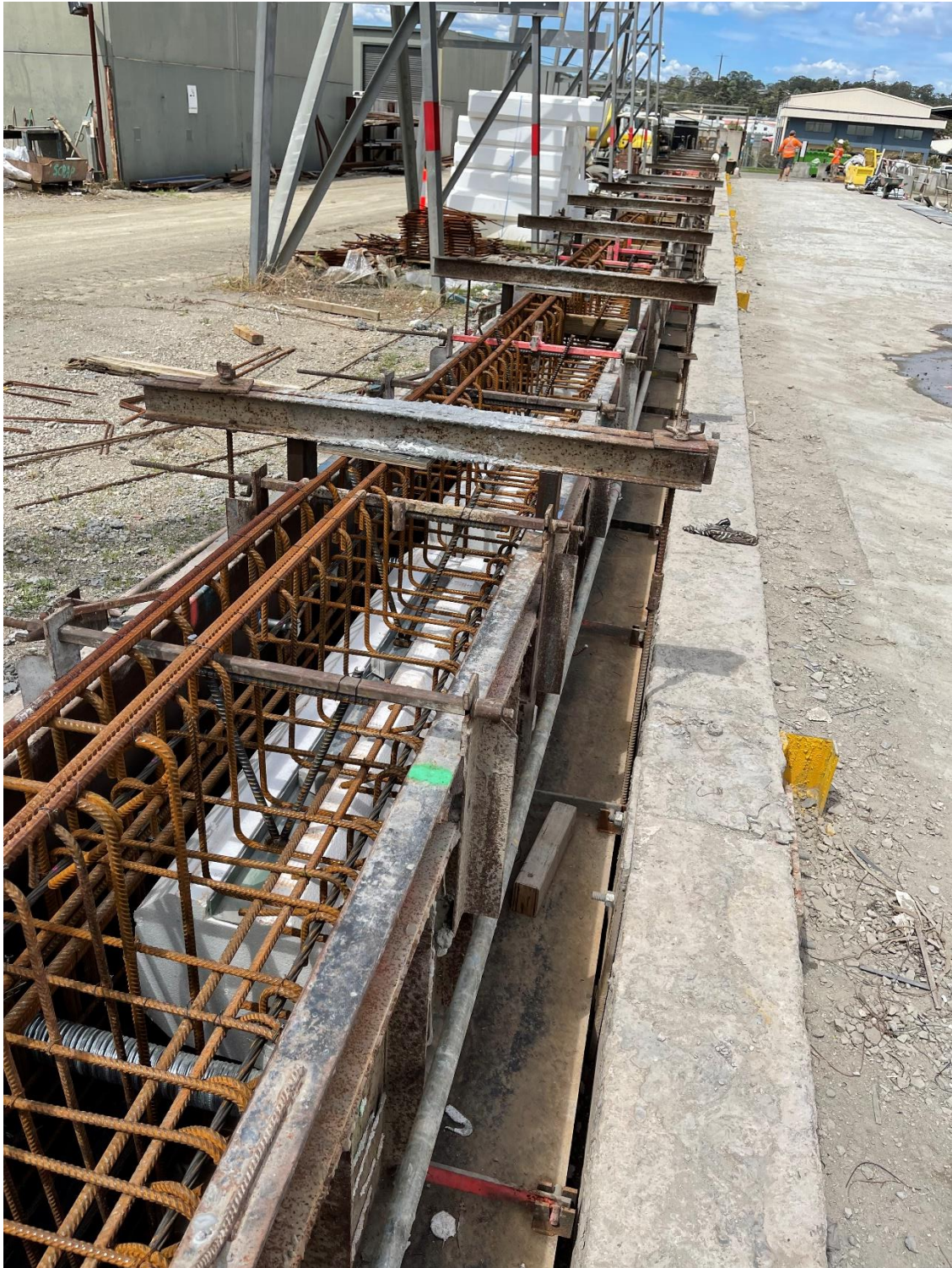
Yetman Road – Moseley Dene Bridge Replacement Project – Prestressed Precast Bridge Planks Being Constructed by Waegar Constructions, Rutherford, NSW
