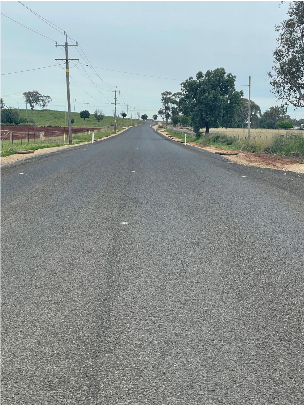
Completion of Primer seal – Ashford Road Wandera South – Southern end of project site
