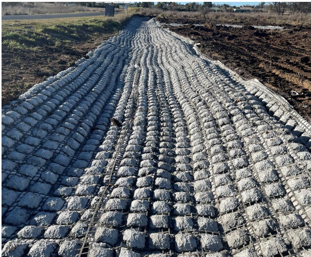
Taylor Avenue Intersection Upgrade Project – Concrete matting installed in open drain
