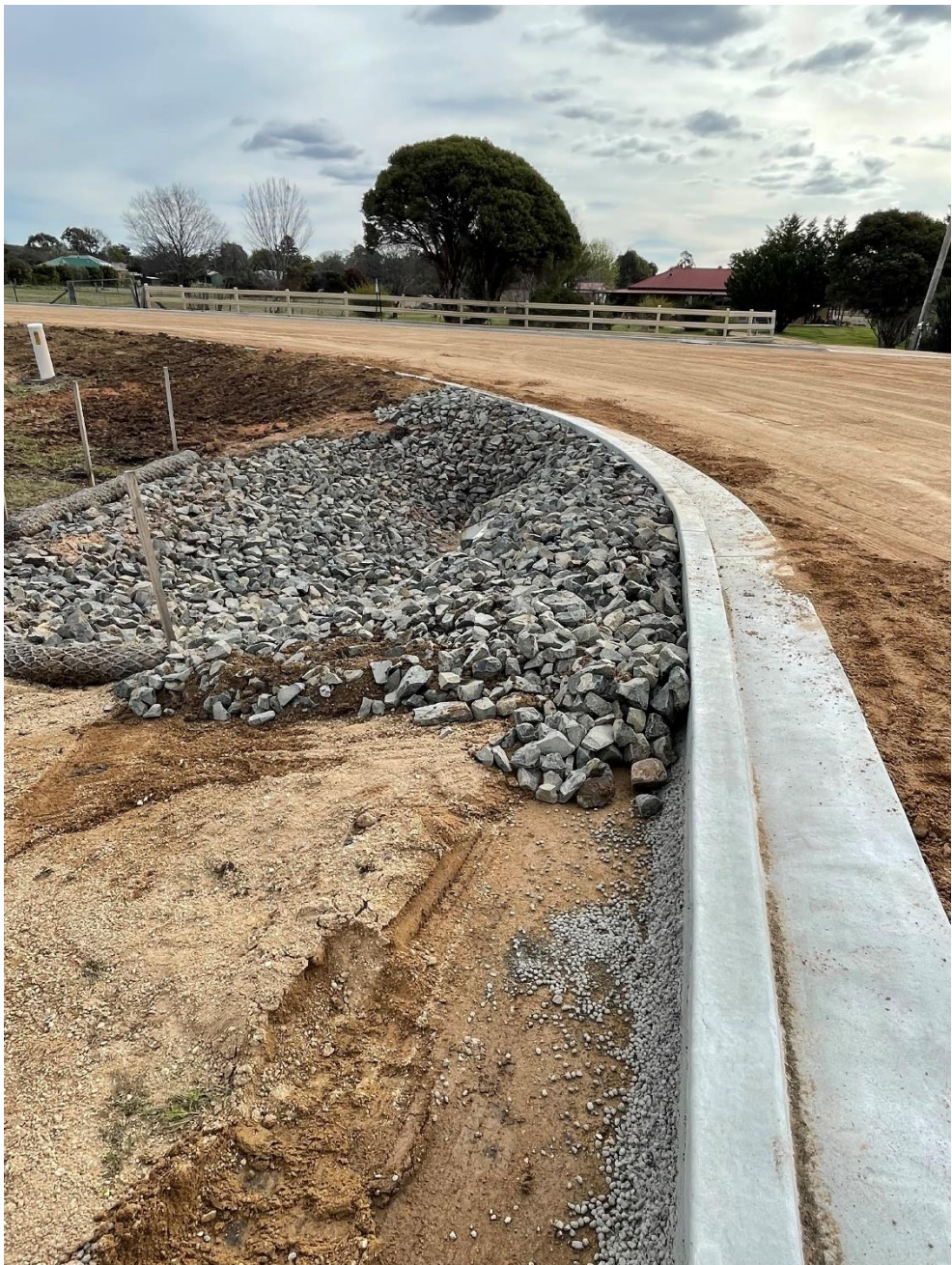
Taylor Avenue Intersection Upgrade Project – Rip-rap rock pitching installed around headwalls for erosion protection
