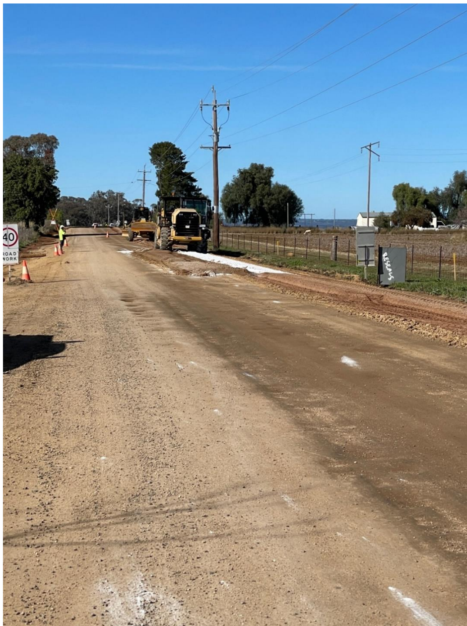
Mixing of subbase shoulders – Ashford Road Wandera South
