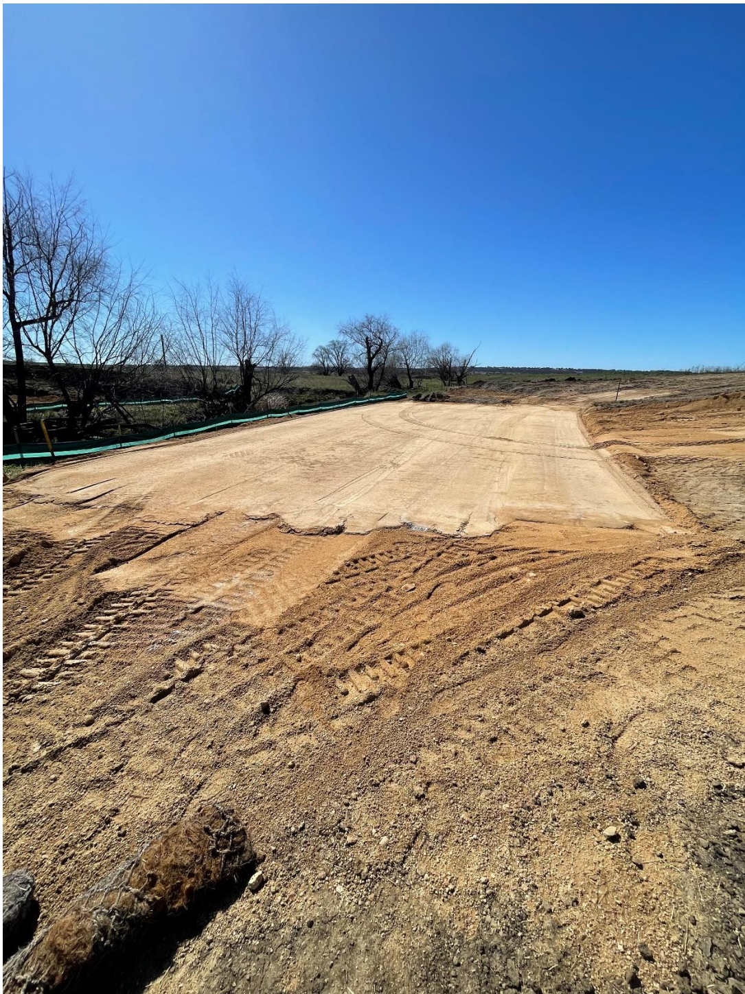
Yetman Road – Moseley Dene Bridge Replacement Project – Working Platform constructed in preparation for the drilling rig to bore the bridge piers
