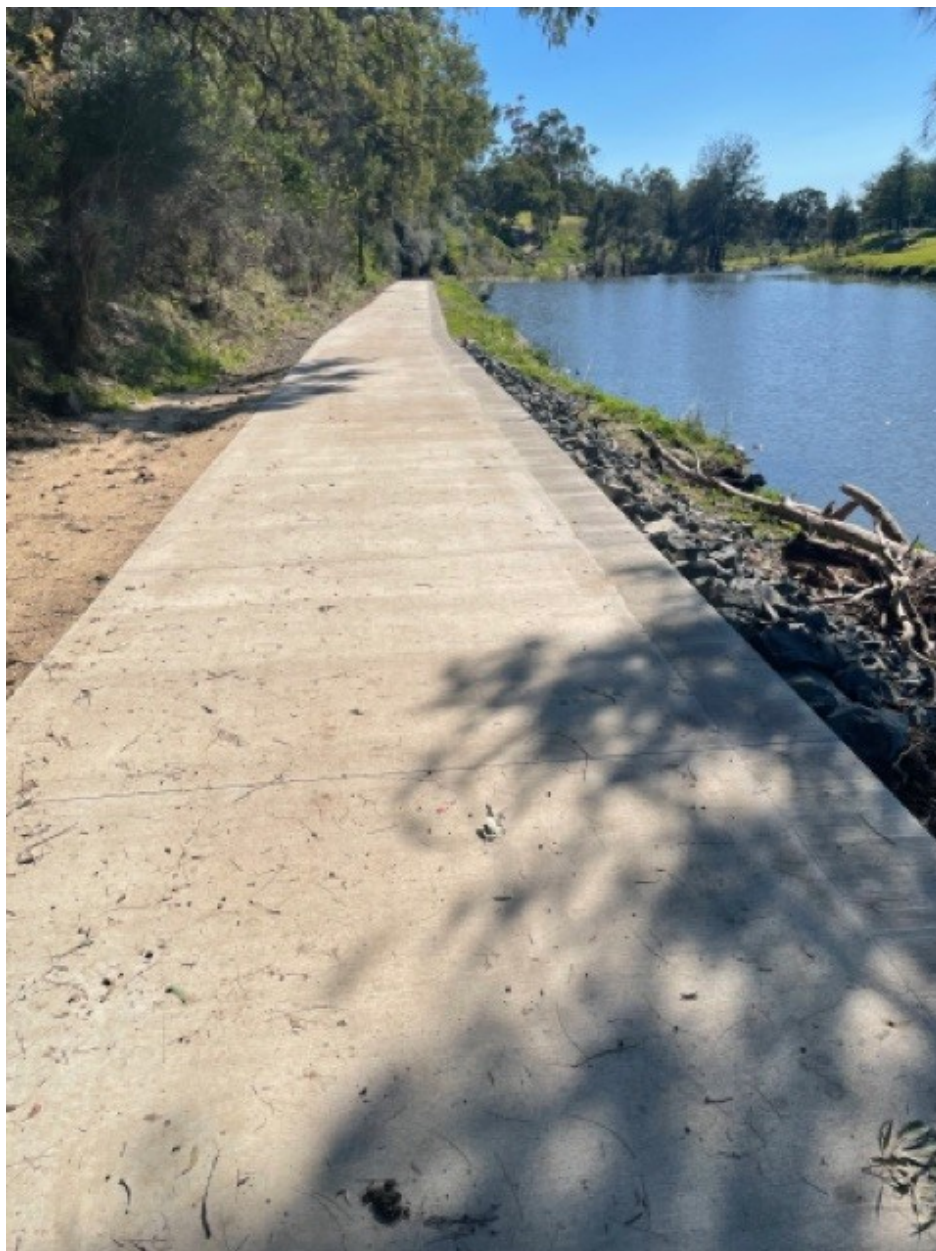
Completed path adjacent Macintyre River with erosion protection completed
