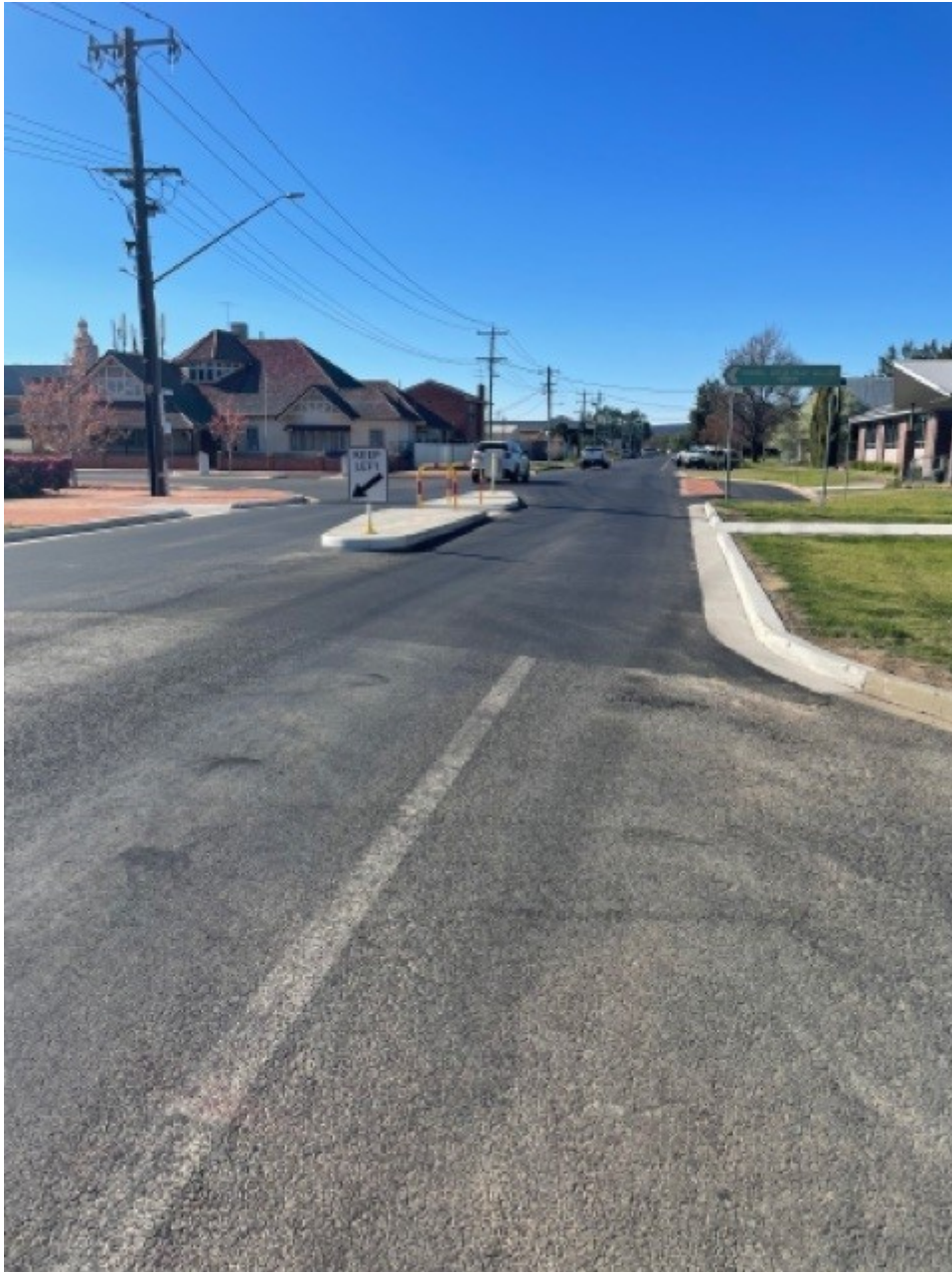
Completed pedestrian refuge and asphalt pavement works
