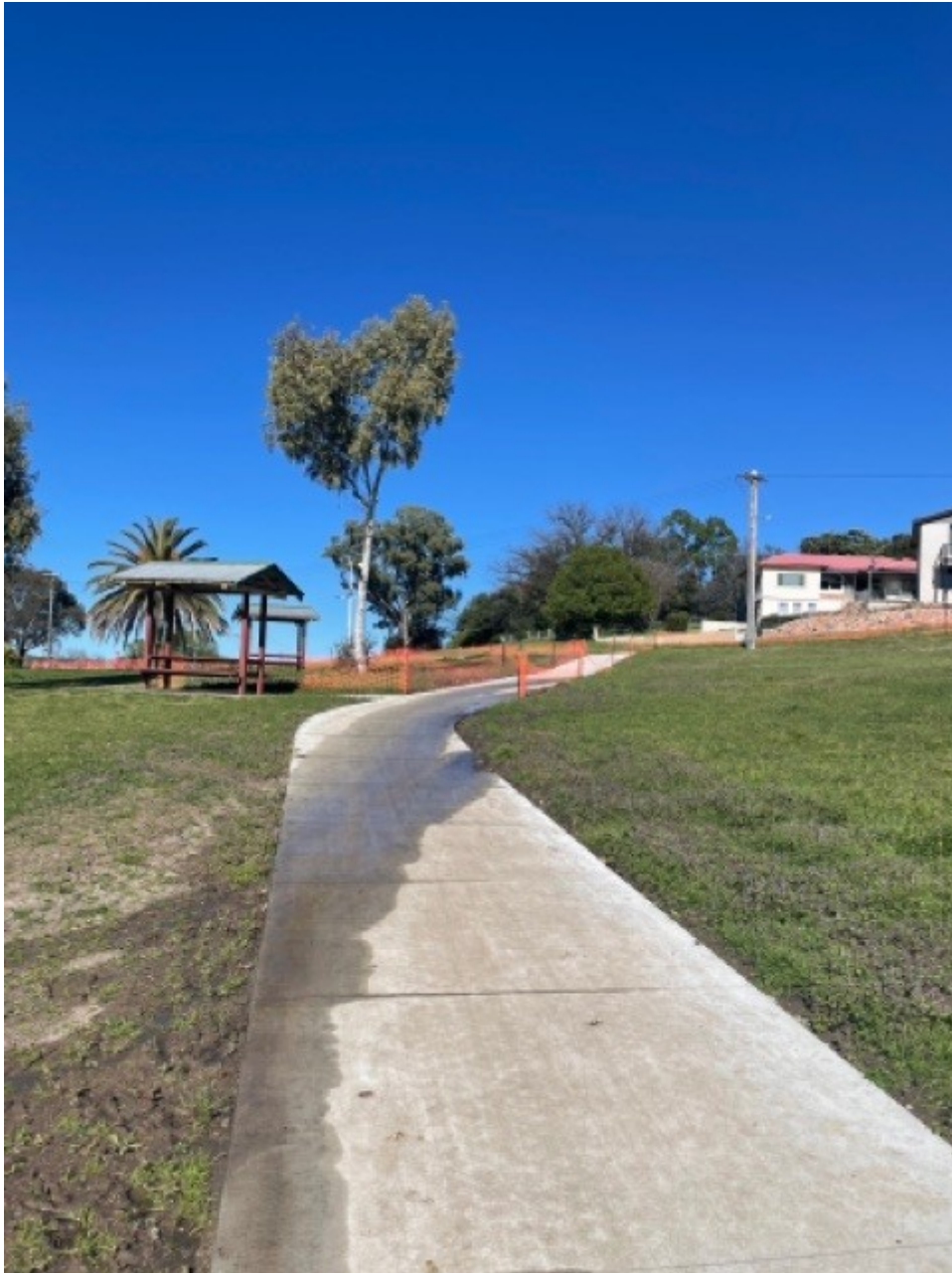
Natural spring water exiting across the newly constructed path
