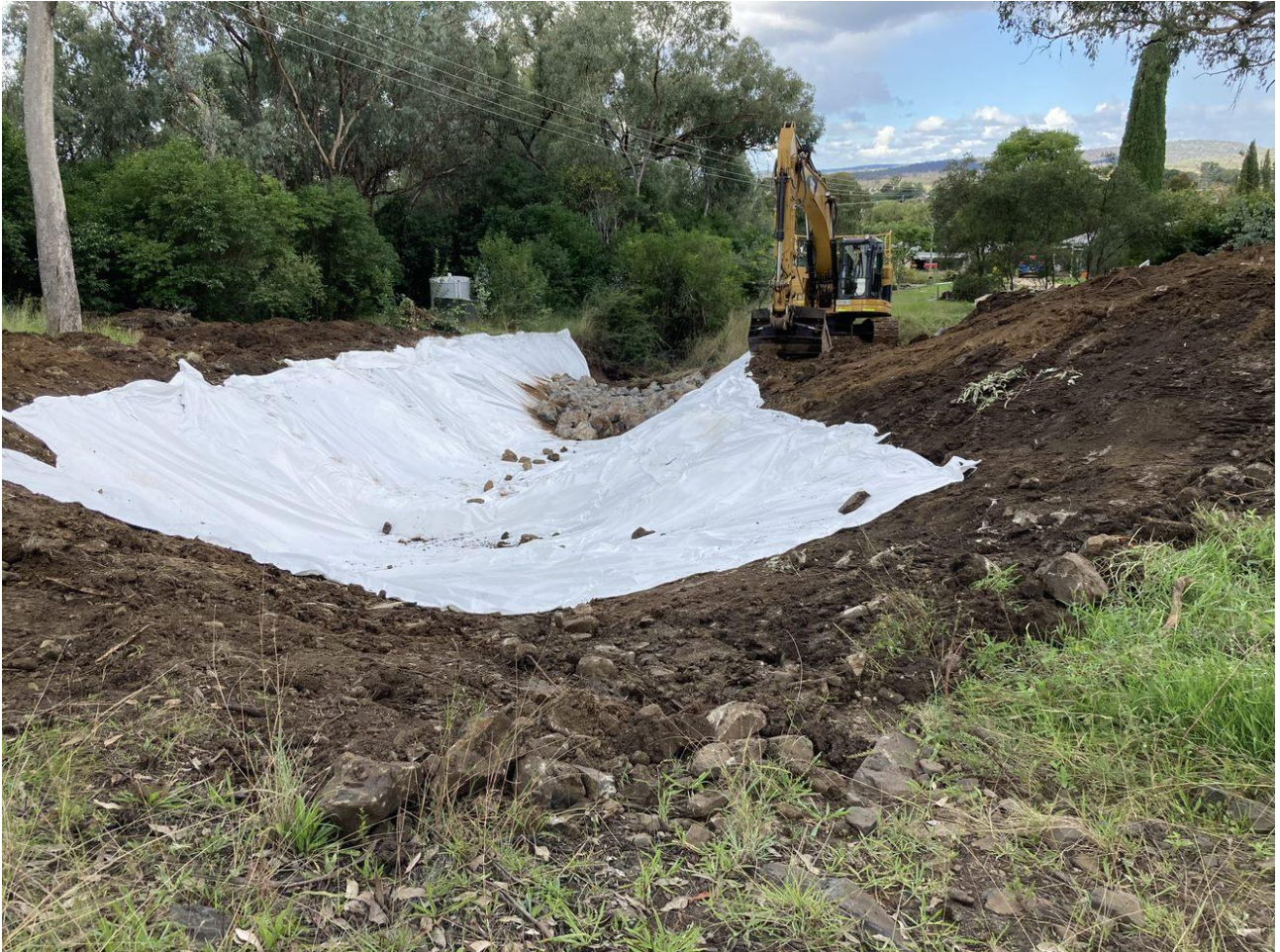
Geofabric lining with rock flume being installed – Froude St Drainage Works
