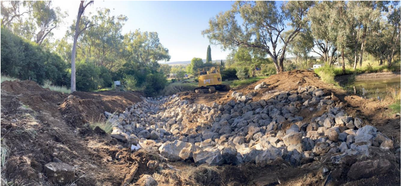
Rock Flume installed and dam wall raised – Froude St Drainage Works
