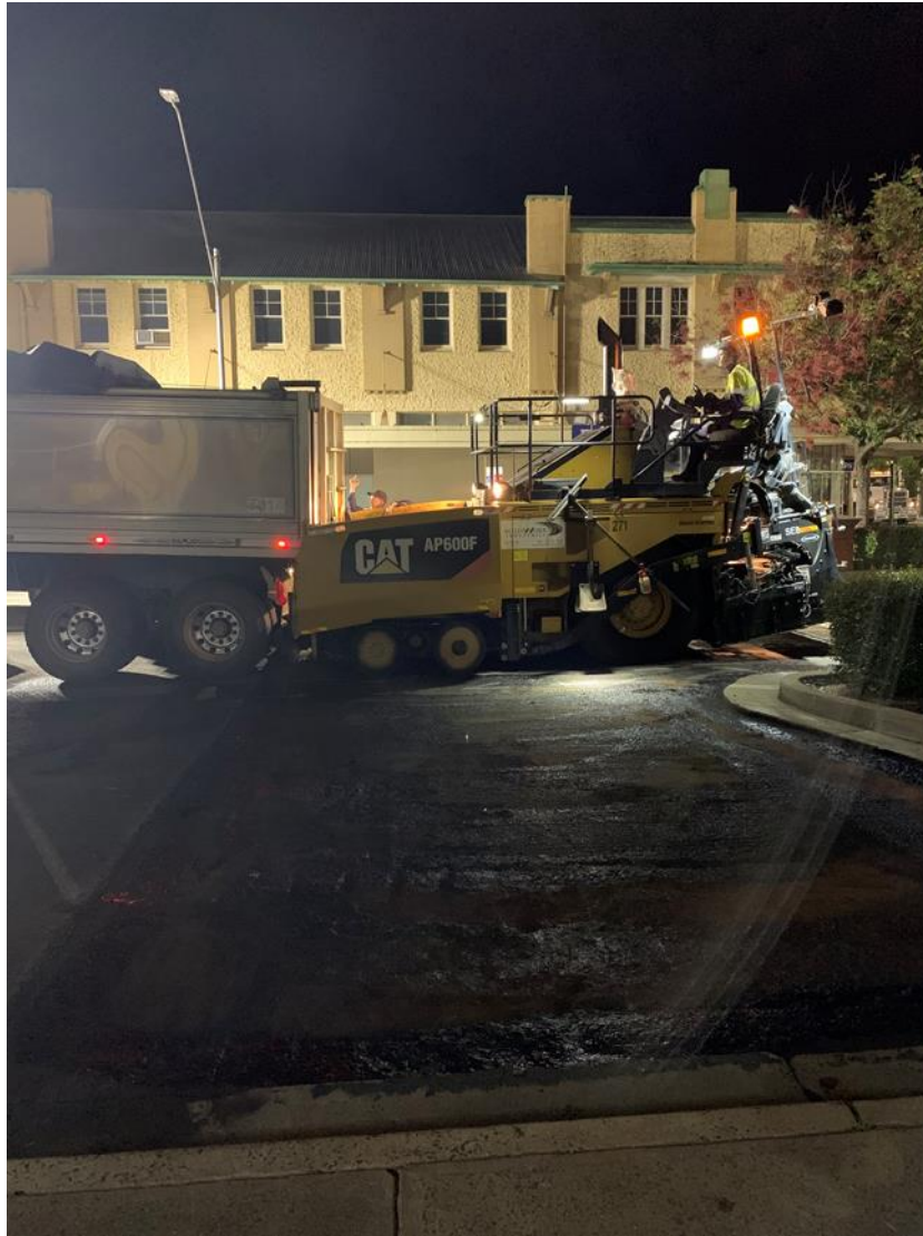
Commencement of asphalt laying in Vivian Street
