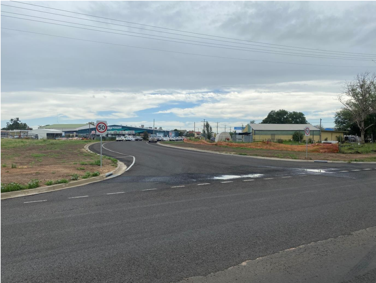
Oliver Street Extension – Pavement Bitumen Sealed and Linemarked
