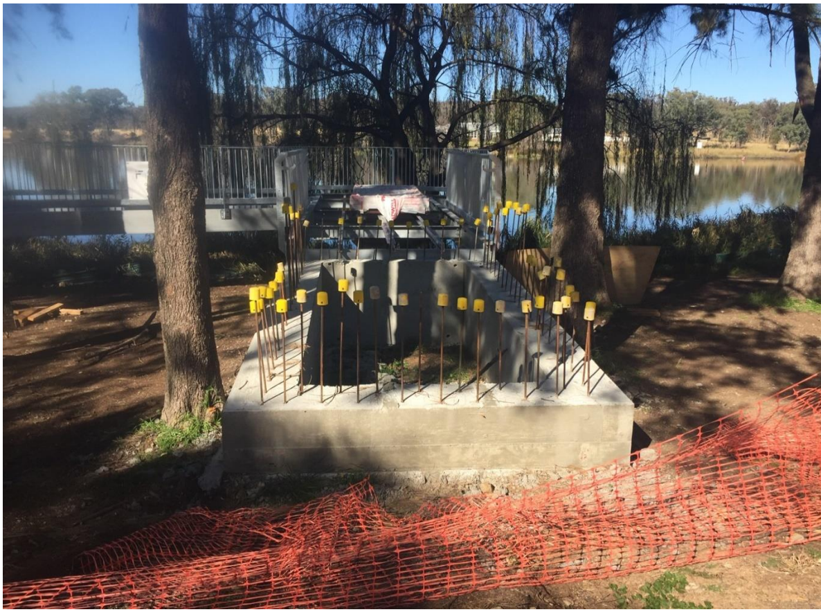
New Boardwalk Abutment – Lake Inverell All Abilities Project
