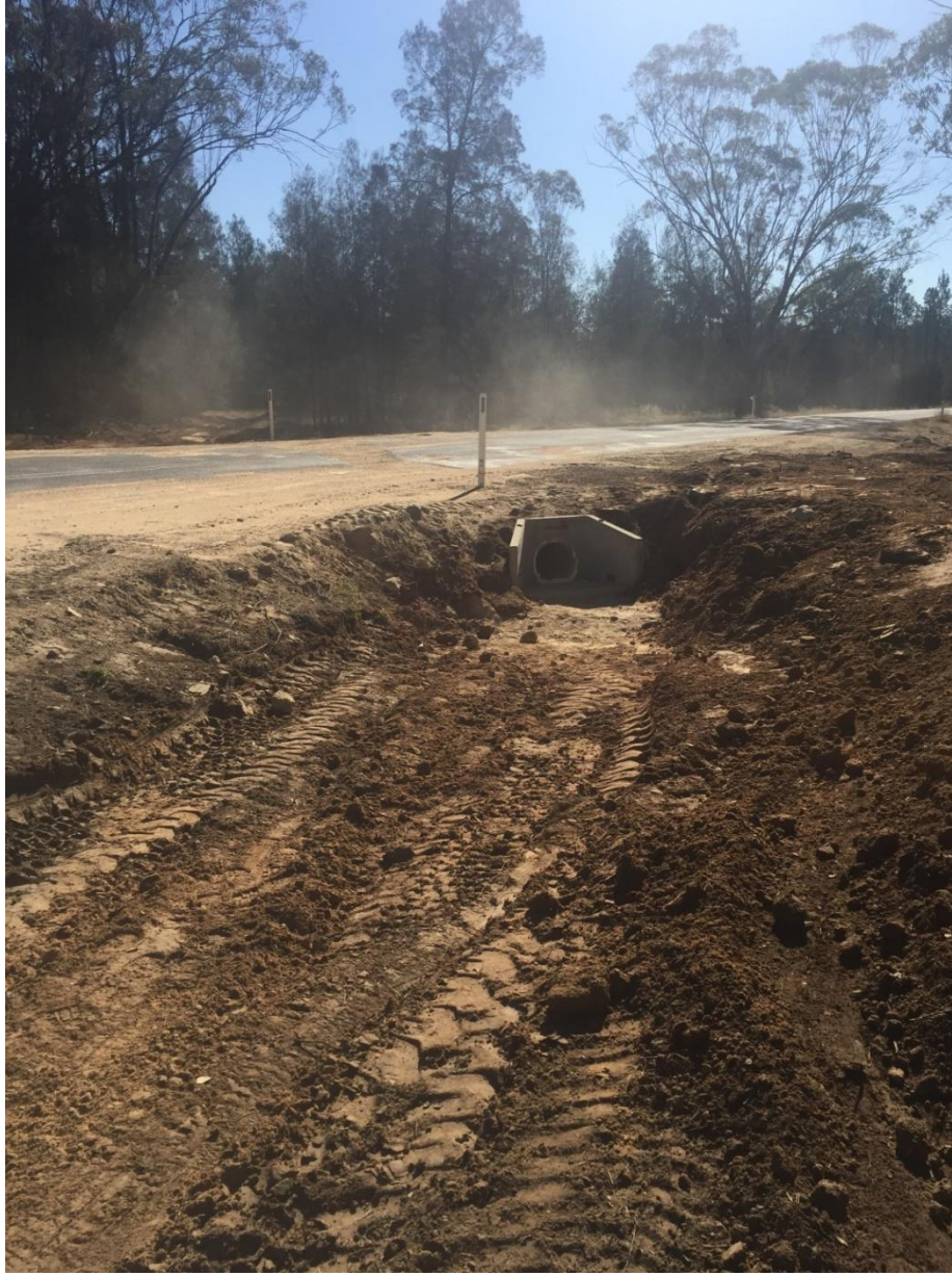
Pipe Culvert Replacement – MR63 “Black Dam” Rehab and Widening Project
