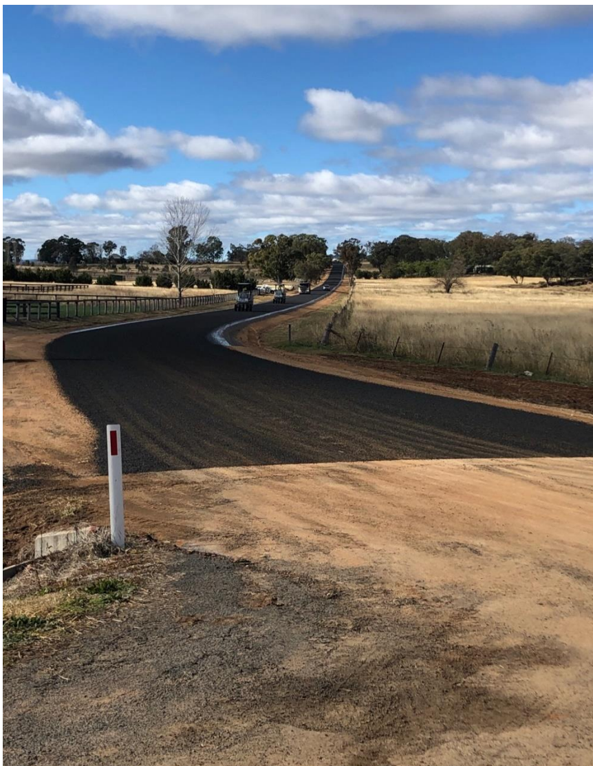
Toms Drive Pavement Rehabilitation – Primer Seal
