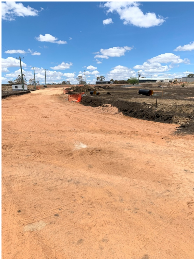
Pavement material placed with drainage under construction– Rifle Range Road Industrial Subdivision
