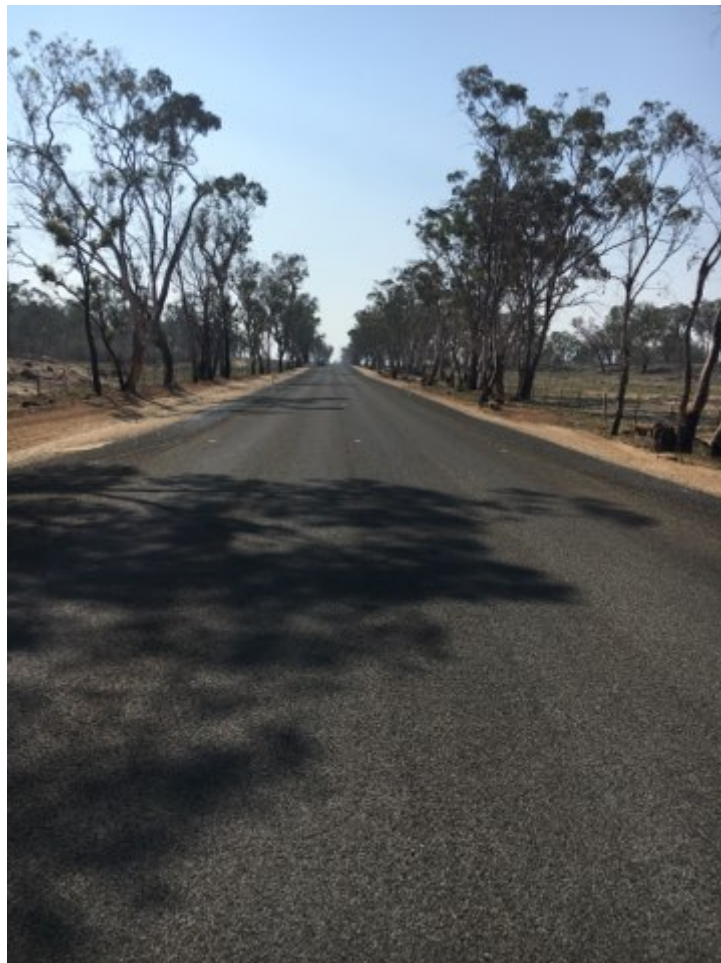
The prime bitumen seal on Stage One MR135 Slurry Gully project
