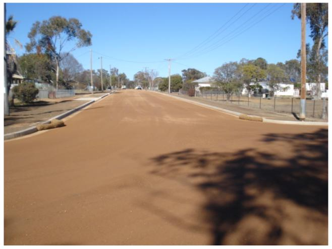
Completion of kerb and gutter and ready for completion of pavement – Wood Street Gilgai
