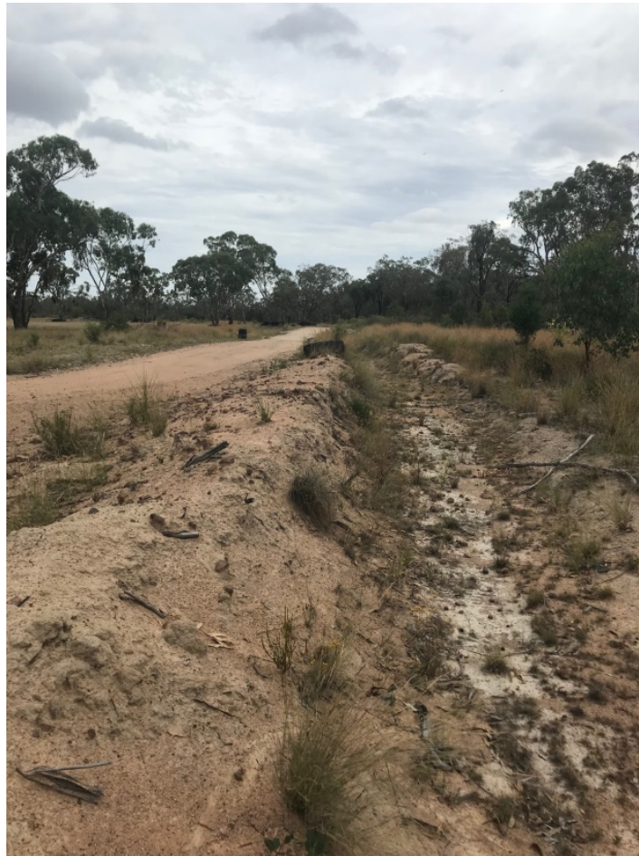
Photograph 6 – A trench has been excavated parallel to the gravel track on the eastern boundary of the reserve. It appears to divert water away from the gravel track.
