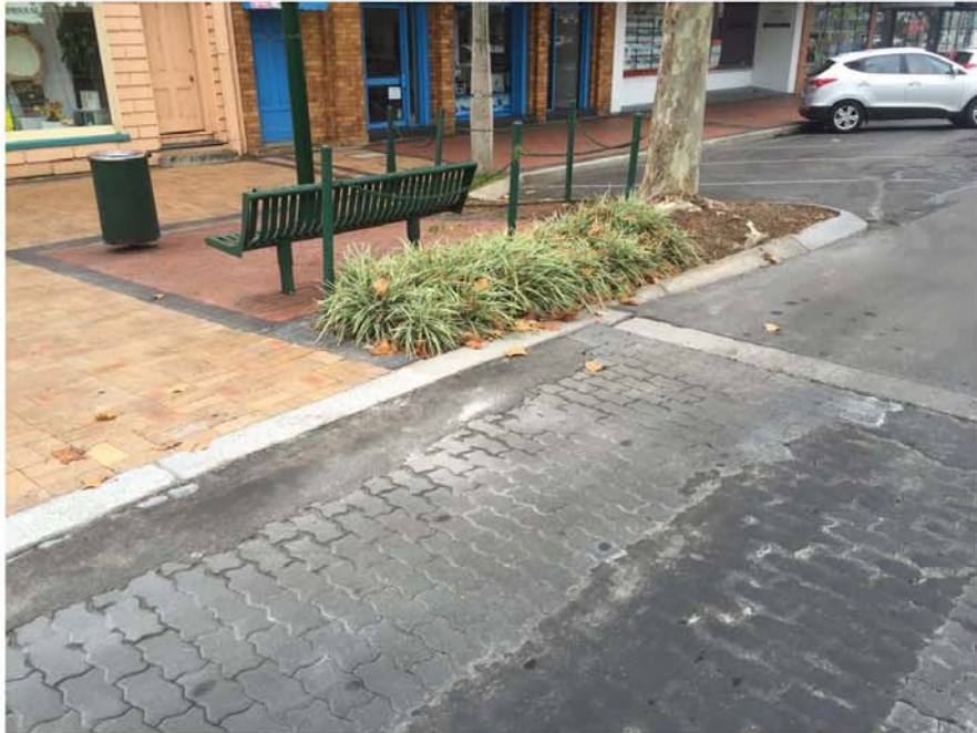
Figure 1 – Superficial repairs to preferred crossing area in Byron Street (near Otho Lane).
