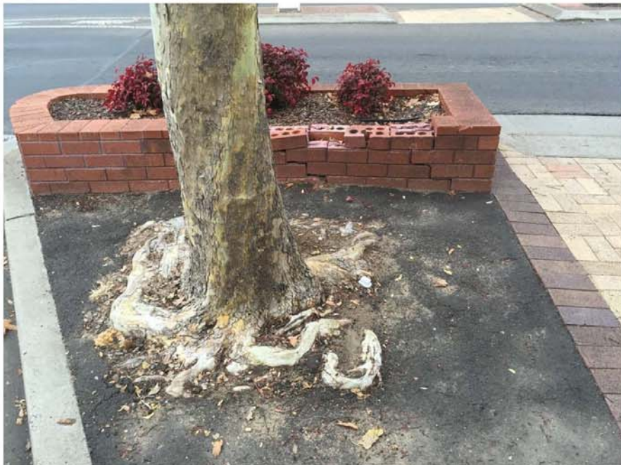
Figure 2 (corner of Byron and Lawrence Street) – Damaged brick garden, cracked kerb and the need to regularly re-lay adjoining pavers. The pavers lead to a pram ramp and crossing point.
