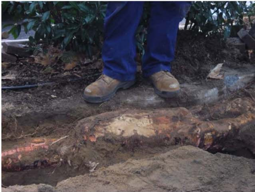
Figure 7 – Close up shot of the root in figure 6 above. Note the bulbous section where the root was cut several years prior to repair similar damage. Roots need to be cut to repair damage, however the Arborists have indicated there is significant risk associated cutting roots of this size.
