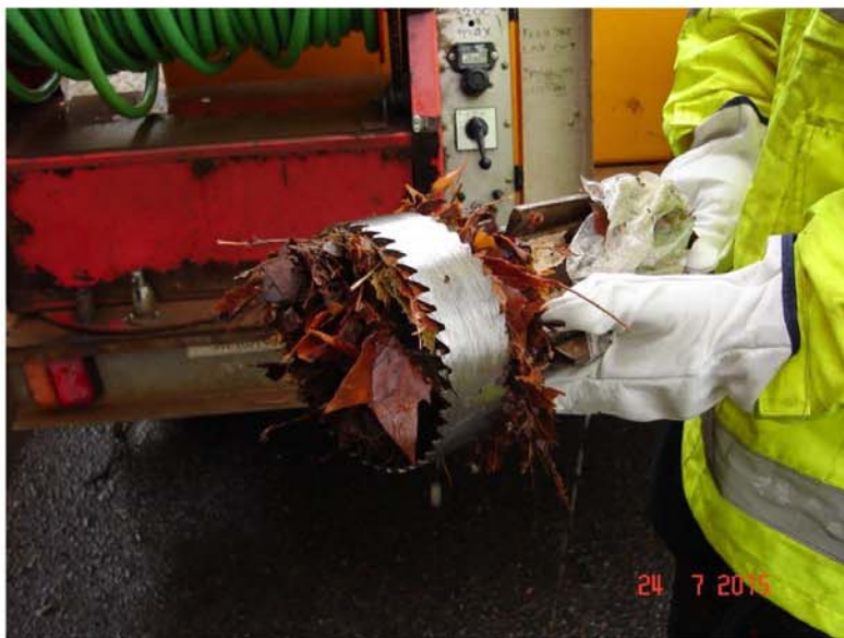
Figure 9 – Small roots and Plane Tree leaves cleared from blocked drain in Figure 8.
