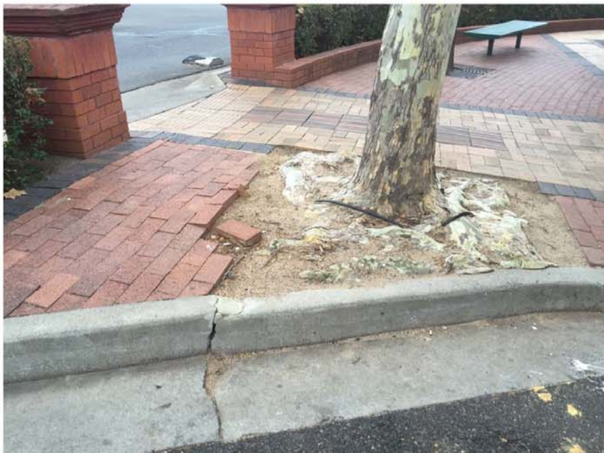
Figure 4 (corner of Byron and Vivian Street) – Cracked kerb and dislodged pavers surrounding Plane Tree. Cracked and damaged kerb adjacent to Plane Trees planted in the footpath is a common occurrence throughout the CBD
