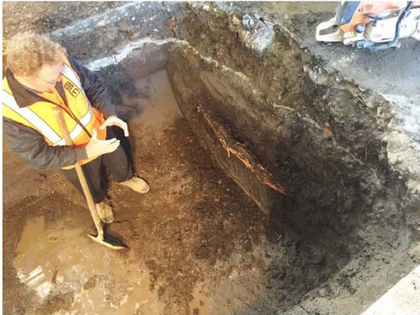
Figure 5 – Excavation for the lift well within the Byron Arcade redevelopment unearthed a Plane Tree root in excess of 100mm in diameter. The lift well is approximately 21 metres from the nearest Plane Tree.
