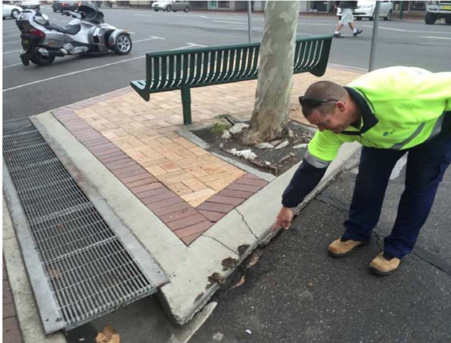
Figure 3 – Bus Stop island in Otho Street being lifted and damaged by Plane Tree root. The island has been lifted to the extent it has dislodged the bolts fixing the grate to the adjacent kerb.
