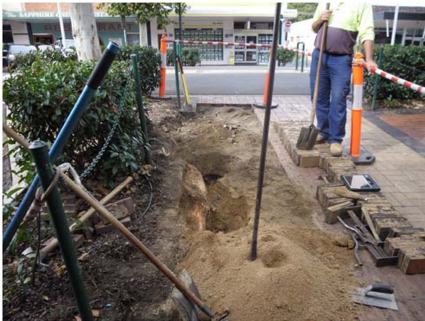
Figure 6 – Large Plane Tree root lifting pavers in walkway at front of Coles metres away from the base of the tree. Note the tree planting in a garden bed.
