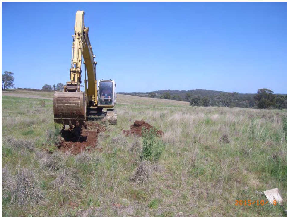
Figure 1 Excavation of test pits
