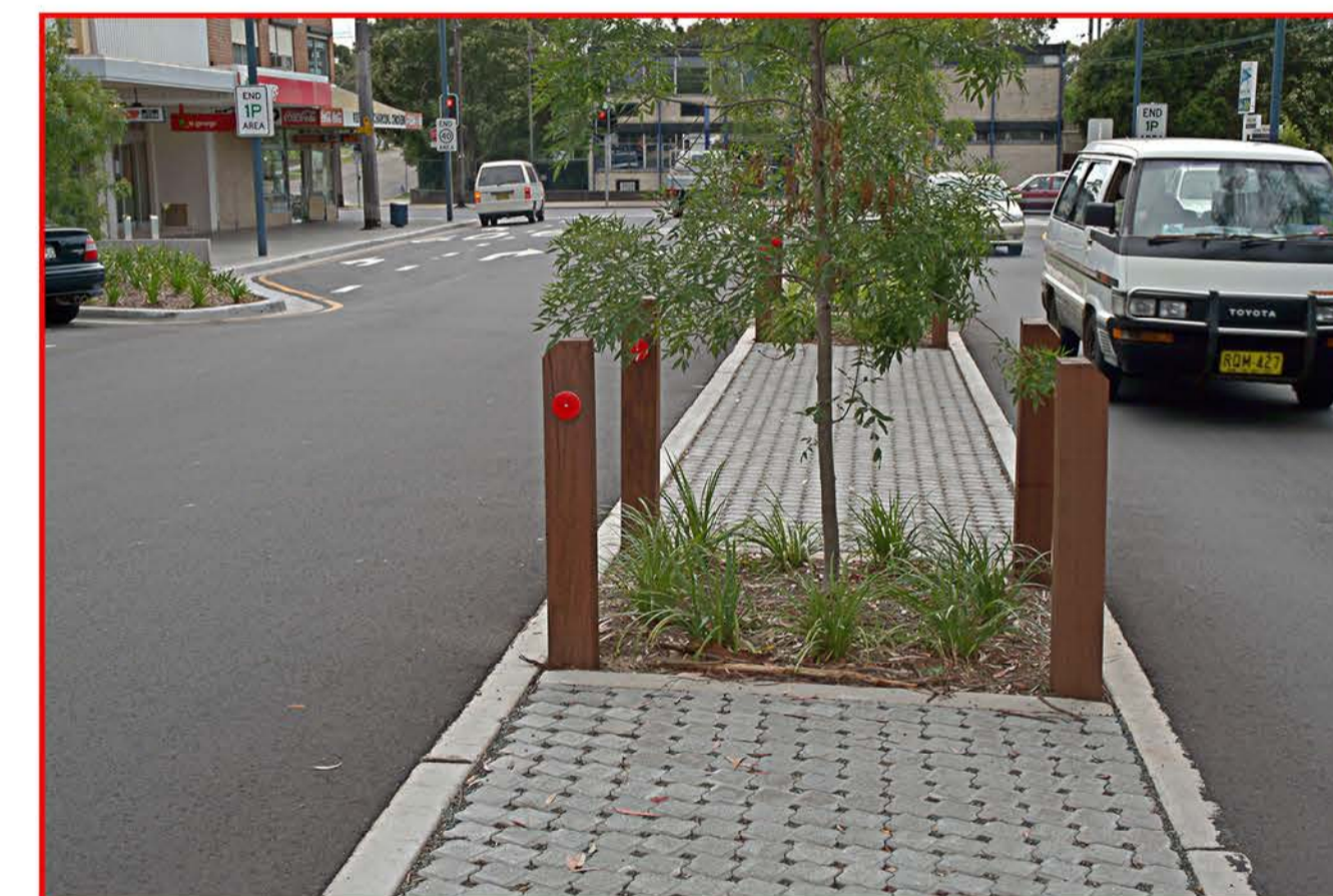
EXAMPLE OF SIMILAR MEDIAN TREATMENT - This median shows permeable paving with flush kerb, like that proposed
