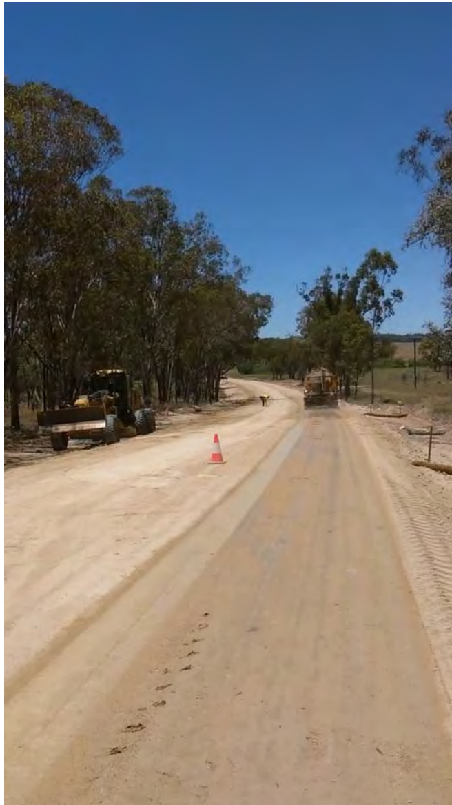
MR 187 Yetman Road Stage 1 - construction of base layer
