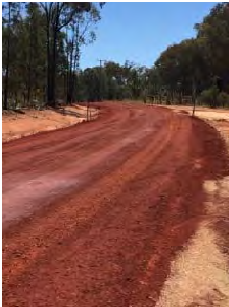
SR 218 Old Stannifer Road - construction of base layer
