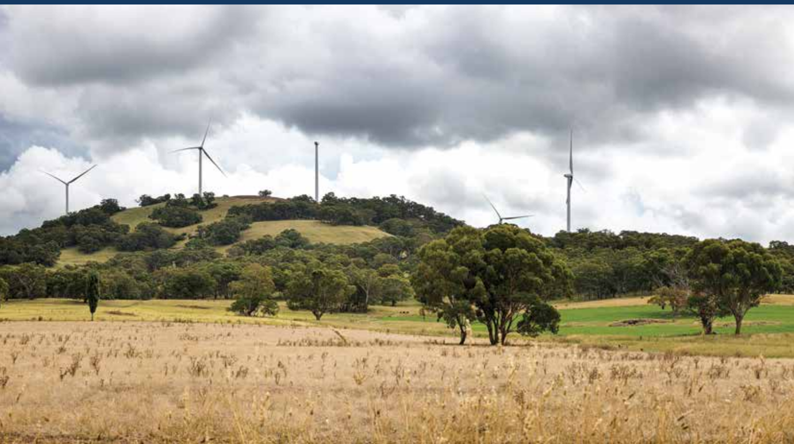
View of White Rock Wind Farm turbines in various stages of installation from Jenkins Road
