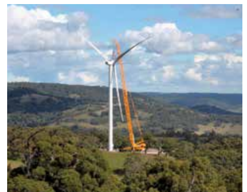
Turbine installations underway.
